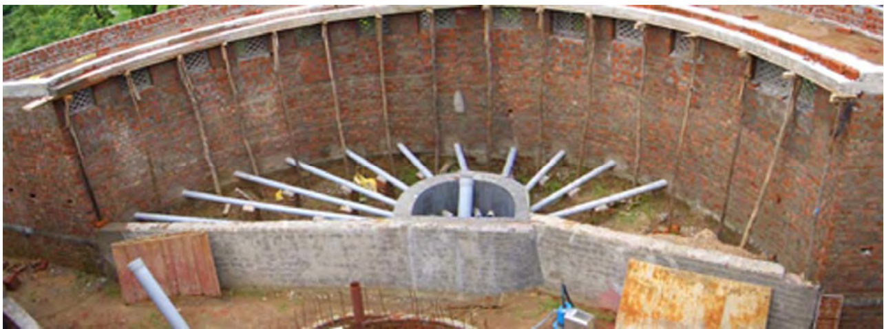
figure 9: Night-soil based biogas plant [clockwise from top left: conceptual sketch of toilet linked biogas system; view of new toilet block; top view of hoppers and biogas plant (under construction); rear view of toilet cabins depicting individual blackwater disposal pipes (before refilling with soil and landscape gardening); picture of “pour-flush” squatting pan with water seal (“P”-trap)]
