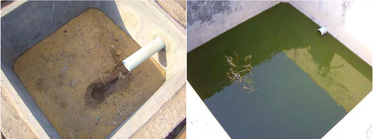
figure 18: Vertical flow organic filter (left) and collection tank for greywater (right)
