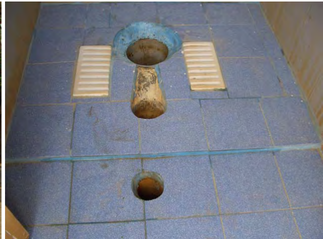
figure 4: ACTS Public Toilet Centre in Rajendra Nagar (left) and squatting slab providing 3 holes for source-separate collection of water used for primary washing hands, urine and feces (right)
