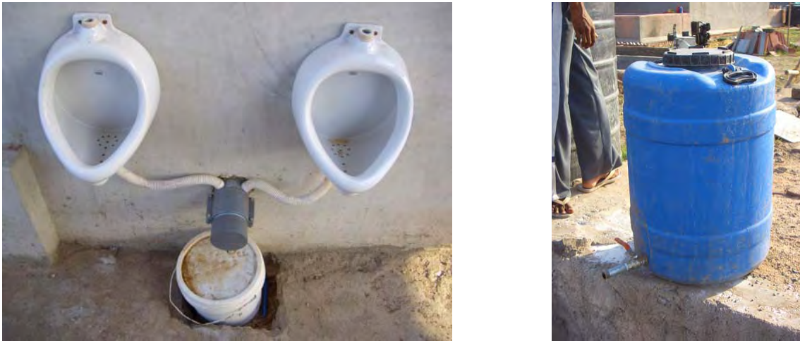
figure 17: Urinals for males and transportable collection tank (left) and storage/hygienisation tank (right)
