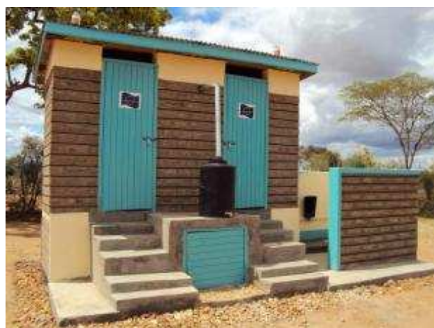
Fig. 3 School UDDT block with two cubicles for boys with urinal on the right and hand washing station in the centre on top of the urine collection chamber at Mwala Primary School near Machakos (source: Johannes Orodí, GTZ-Kenya, Oct. 2009).
