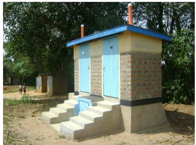
Fig. 5 Newly finished block of two school UDDTs in Western Province. Old pit latrines are visible in the background (source: Moses Wakala, GTZ, April 2009).
