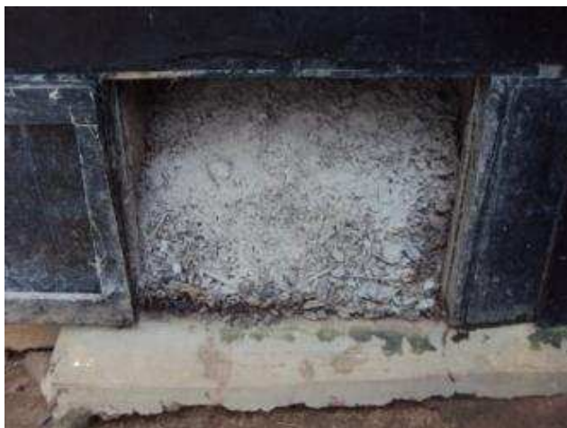
Fig. 8 Faeces vault of UDDT with ash-covered dried faeces (source: Laura Kraft, GTZ, June 2010).
