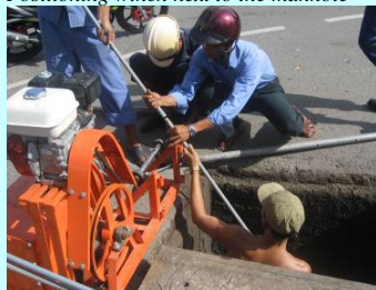
One of two slings is pulled through the Sewer, between manholes
