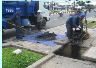
Remove sludge from sewer
