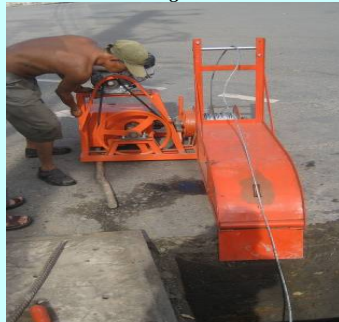
Positioning winch next to the manhole
