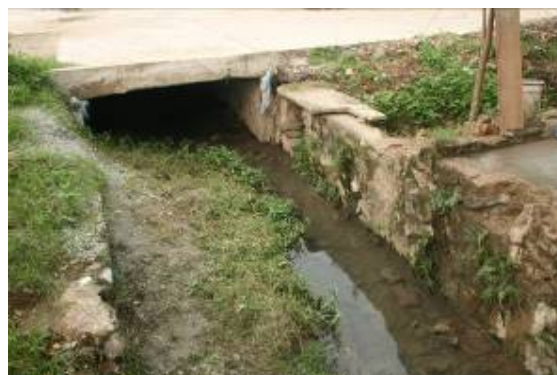
The wastewater from the beer factory flows directly into the urban wastewater drainage system
