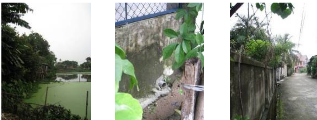
Figure 5-6 Household drains are mostly covered or “half covered and half open”
