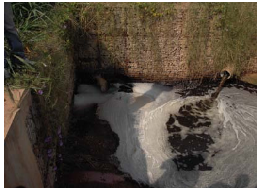
Figure 4-8 : Foamy black effluent from Dompouse FSTP discharged into the Wewe River. (photo: Anselme Vodounhessi)
