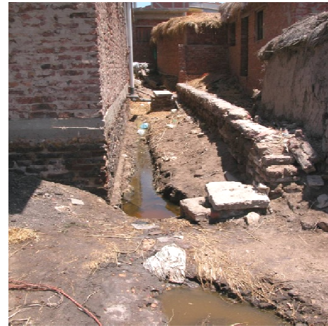
Fig. 5: Wastewater in the streets of El-Moufty El-Kobra before the project in 2002, a common situation in the villages of the Nile Delta (source: GIZ; 2002).
