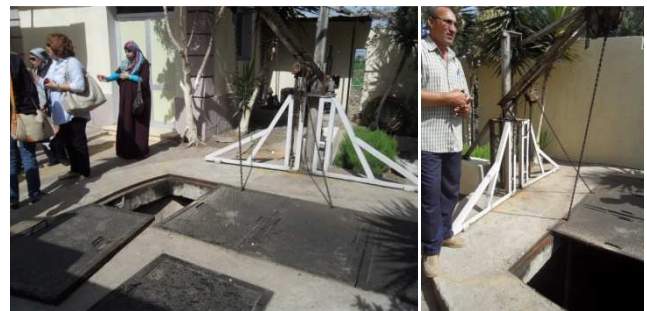
Fig. 7: Pumping station of El-Moufty El-Kobra. On the right picture: Head of the CDA (source: N. Stuber; 2010).
