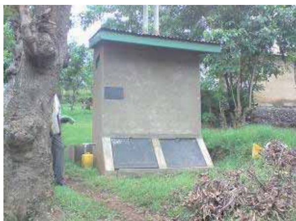
Figure 3 The slanted trap door serving the important role of absorbing heat from the sun.
