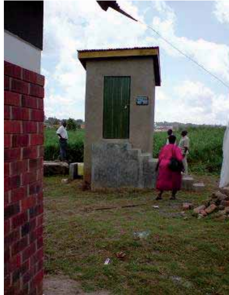
Figure 8: An EcoSan latrine located just 30 m from the raised pit latrine in figure 7. The raised pit latrine can be adapted to EcoSan by modifying it.
