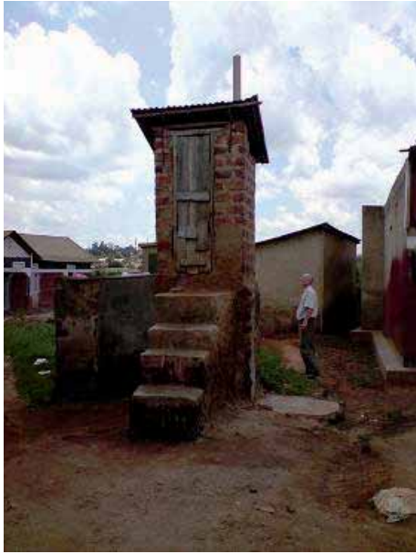
Figure 7: The EcoSan latrine imitation? No, this is the raised pit latrine, near the EcoSan latrine, figure 8.
