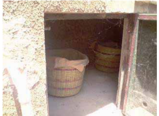
Figure 6 A clean vault using locally made baskets. Note the filled basket on the side.
