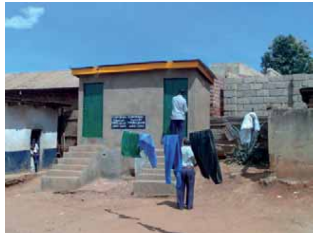
Figure 14 A well exposed EcoSan. However, there is a wall coming up at the back, which will reduce the solar radiation.
