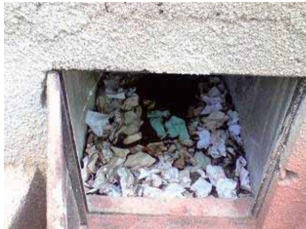
Figure 2: Poor operation and maintenance of the EcoSan at Kawala SS. Note the use of newspapers for anal cleansing and almost no ash applied.
