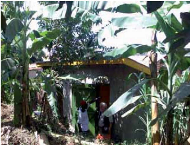
Figure 13: A leafy environment reduces the temperatures in the EcoSan latrine, which may reduce pathogen die-off.
