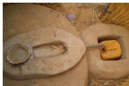
The fossa alterna with urine diversion
