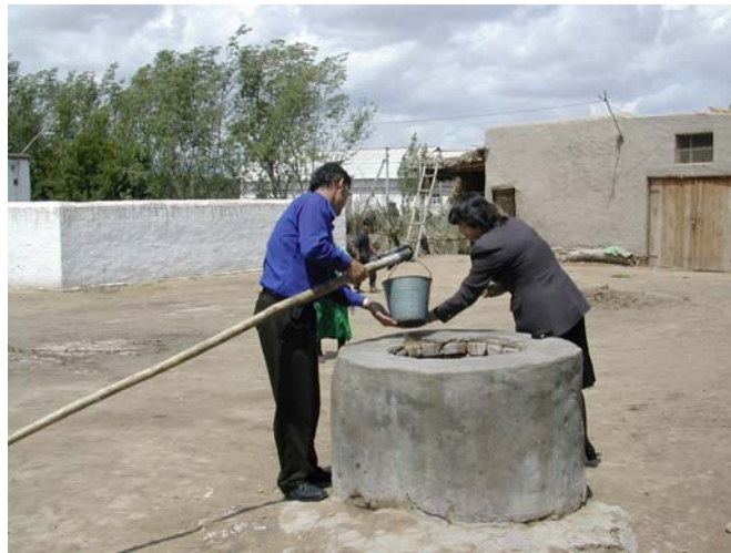
Figure 3.7 Dug well with brick wall providing minimal protection
