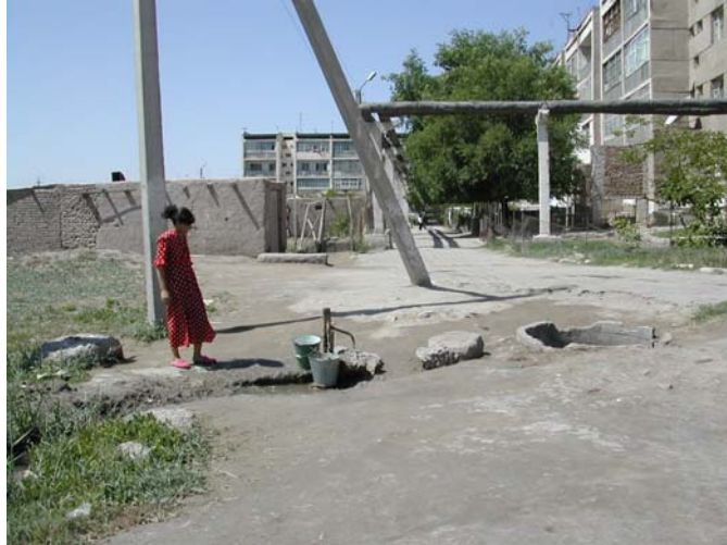
Figure 3.6 Piped water standpipe on the street
