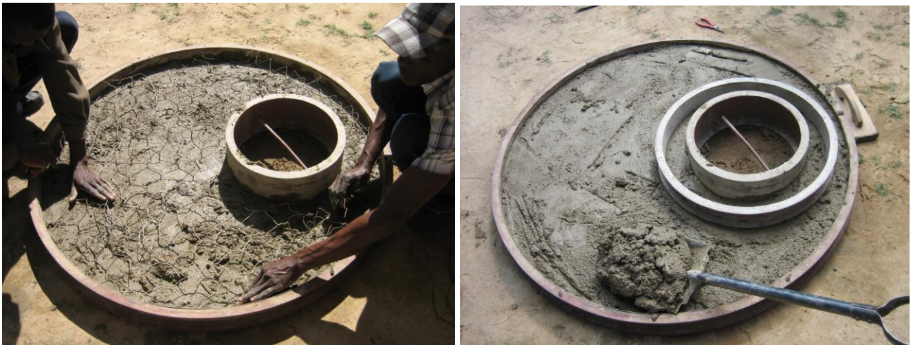
The 1.2m diameter cover slab being made
