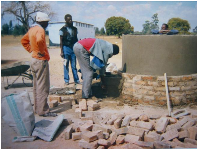
School tanks being built as part of an Mvuramanzi Trust project.
