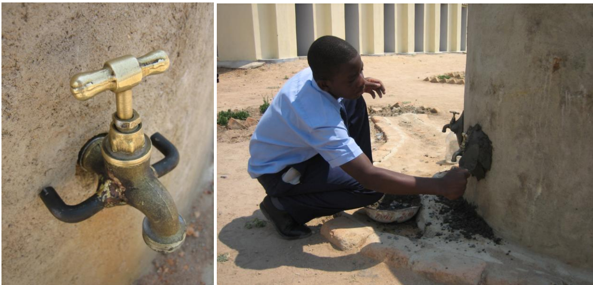
The tap is fitted and the securing mortaring being made
