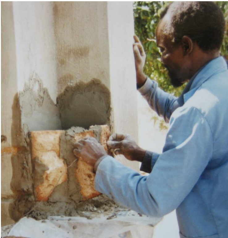
Building the hand washing device on a VIP toilet
