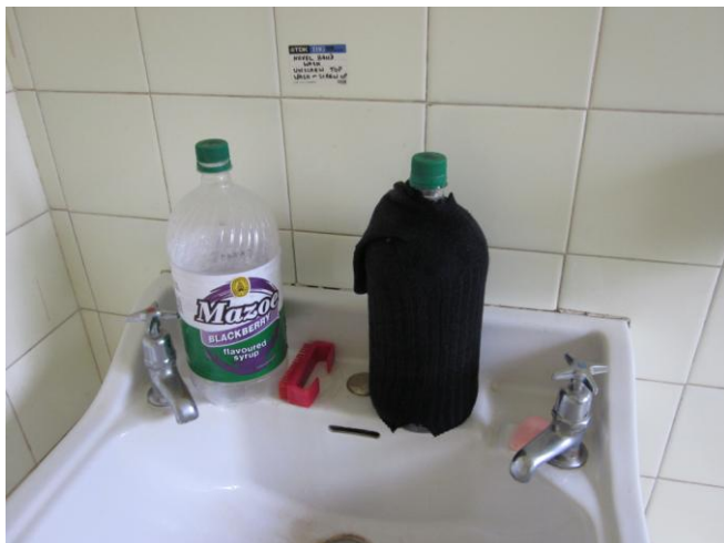
Two hand washing bottles set up on a hand washing basin. The taps do not deliver water, but the bottled do. One is covered with a dark shade cloth to prevent algae growing in the bottle.
