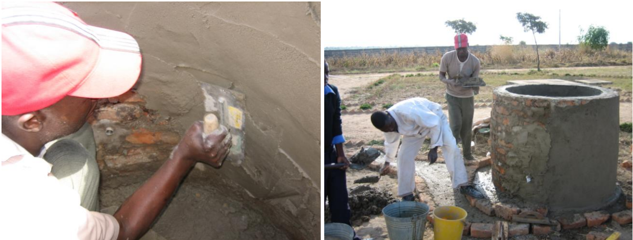
The walls of the tank are plastered inside and outside
