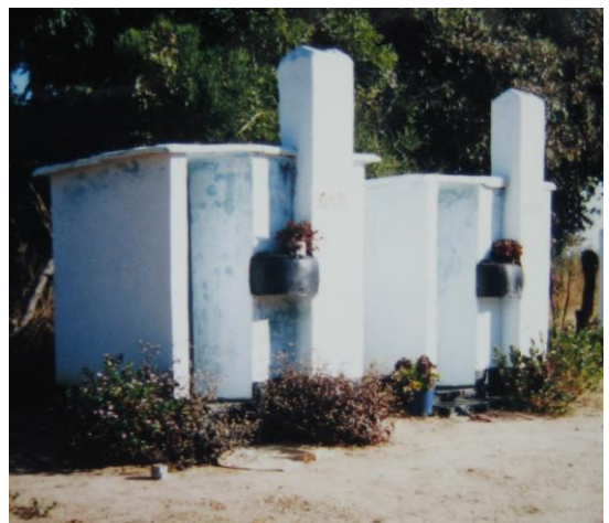
Building the hand washing device on a VIP toilet
