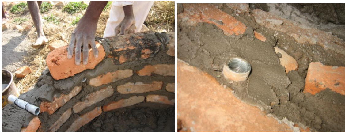
After the pipes are inserted in the cement mortar the brick wall is continued up.
