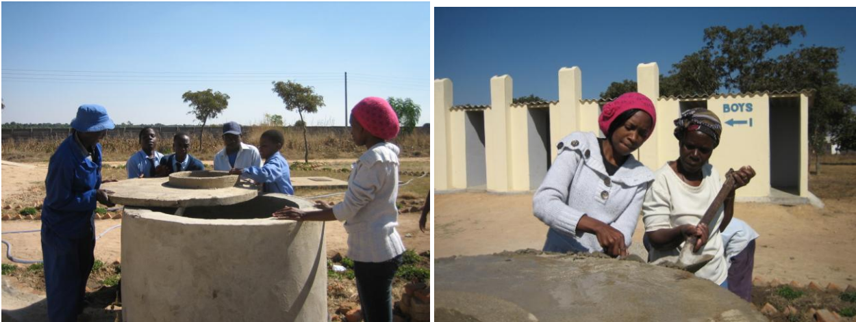
Adding the concrete cover to the tank
