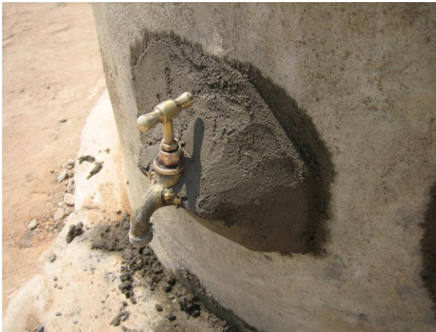
The tap mortared in position. The mortaring was undertaken by a student at the school. Students have been taught how to make toilets and hand washing devices in Epworth
