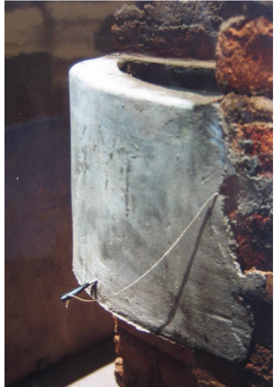
Building the hand washing device on a VIP toilet
