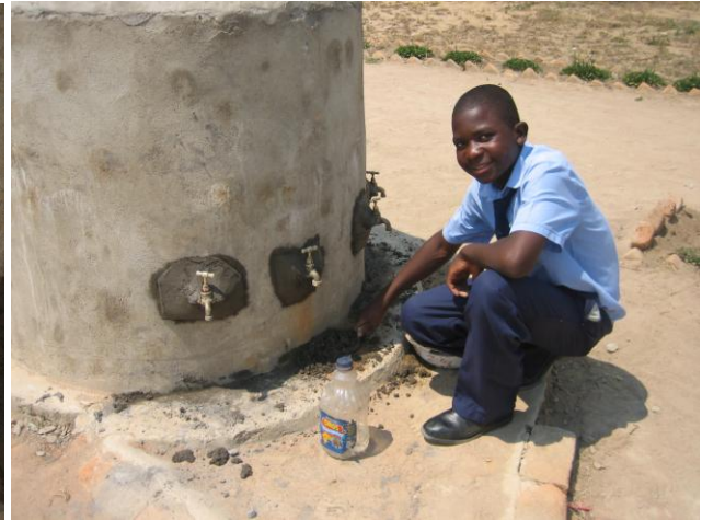
The tap mortared in position. The mortaring was undertaken by a student at the school. Students have been taught how to make toilets and hand washing devices in Epworth
