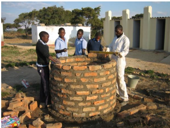
The brick tank is built up to just over one metre high. The actual size of the tank is not specific. Larger tanks with greater capacity can be built.
