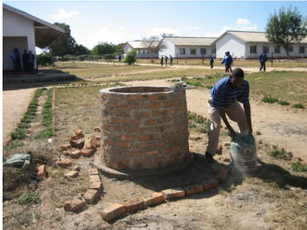
The brick tank is built up to just over one metre high. The actual size of the tank is not specific. Larger tanks with greater capacity can be built.
