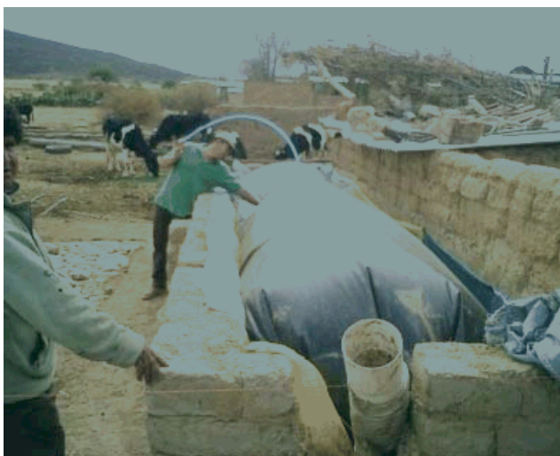
Figure 2: Bag digester in Bolivia. Source: www.tecnologiadesarrollo.tk
