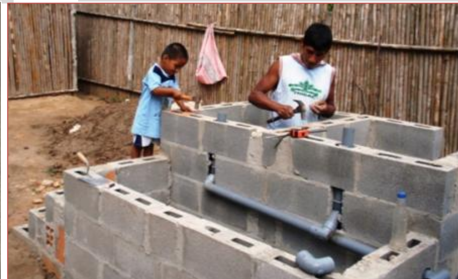
PHOTO 13: Building site with installed urine pipe
