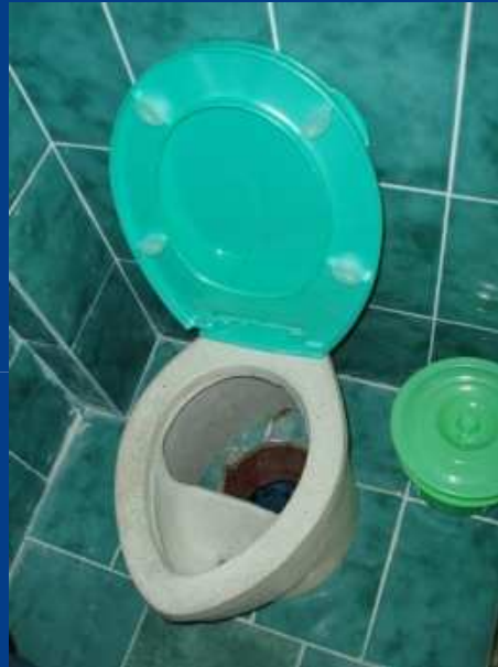
Made of concrete (Mexican mould) by company
