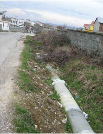
Figure C.50: Concrete wastewater pipe in Rrushkull (Niebel 2012)
