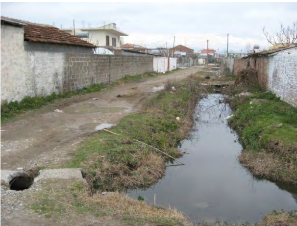
Figure C.52: Open sewer for rainwater and wastewater collection in Rrushkull (Niebel 2012)
