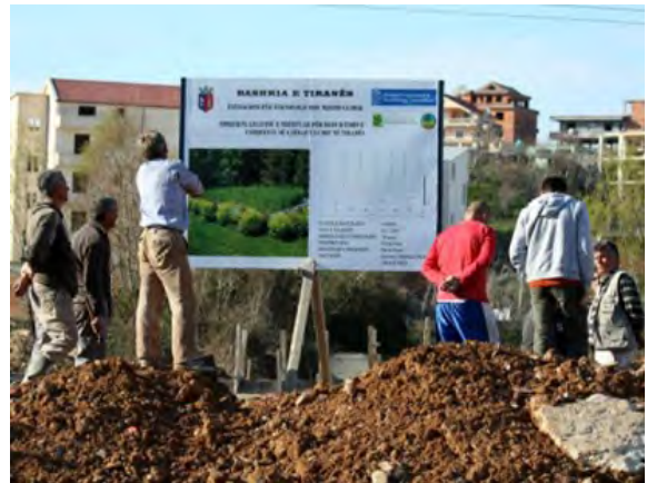
Figure 5.12: Construction side of the research plant at Tirana River (LWE 2011)
