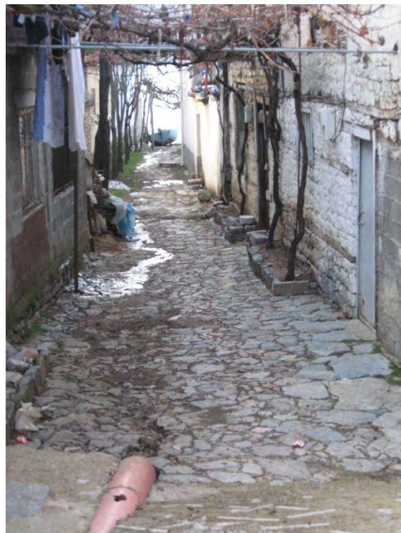
Figure C.43: Discharged water runs directly into the lake (Niebel 2012)
