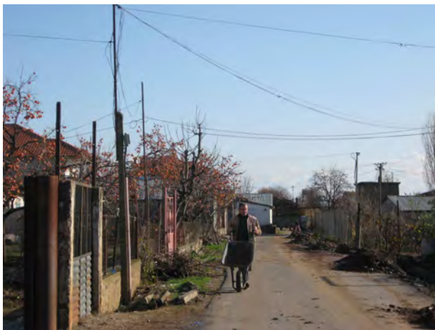
Figure C.3: Asphalt street in Dober (Niegel 2011)
