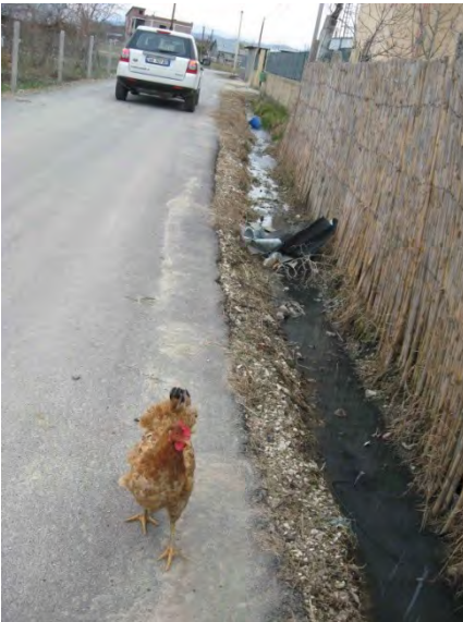
Figure C.56: Open sewer in Hamallë (Niebel 2012)
