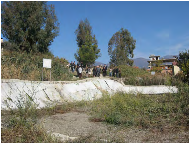
Figure 5.7: Horizontal filter bed with only few vegetation in November 2011 (Niegel 2011)
