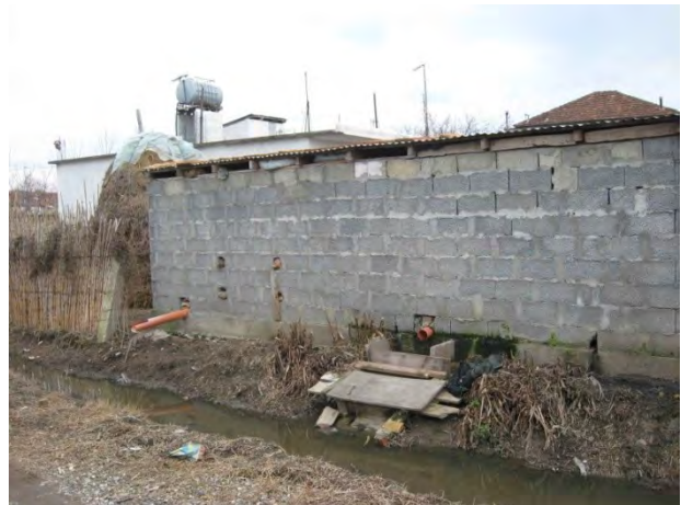
Figure C.53: Pipes from the private yard lead wastewater into the open sewer in Rrushkull (Niebel 2012)
