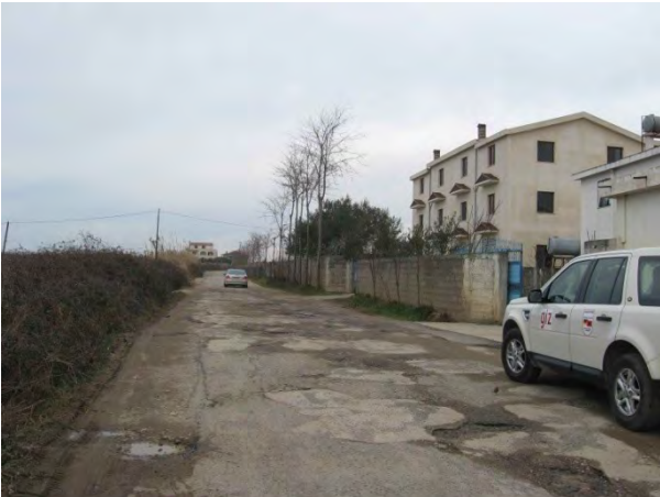
Figure C.46: Village Perlat, main streets is mostly damaged (Niebel 2012)
