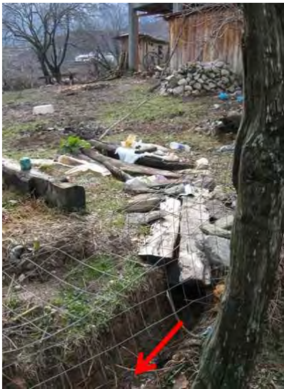
Figure C.34: Free wastewater discharge in the garden (Niebel 2012)
