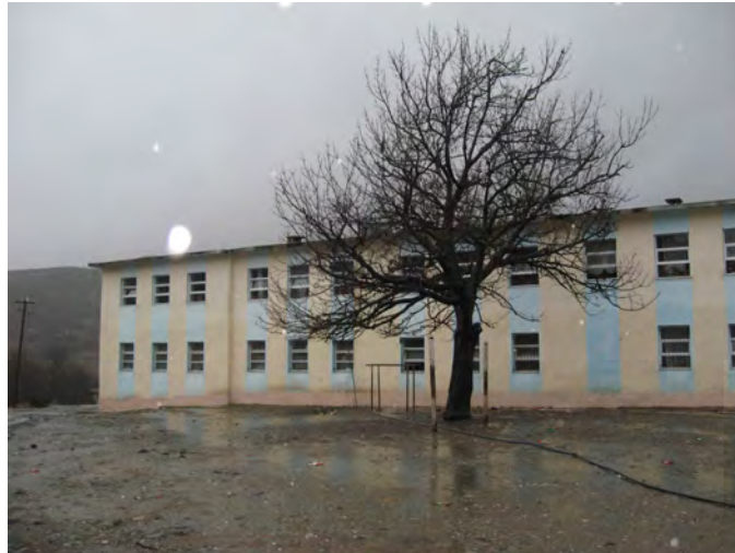
Figure C.9: School for 380 students in commune Qelez has no water supply (Niebel 2012)
