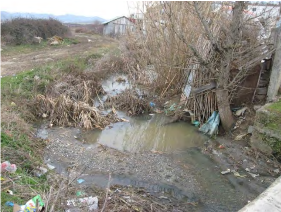
Figure C.54: Wastewater collector in Hamallë (Niebel 2012)
