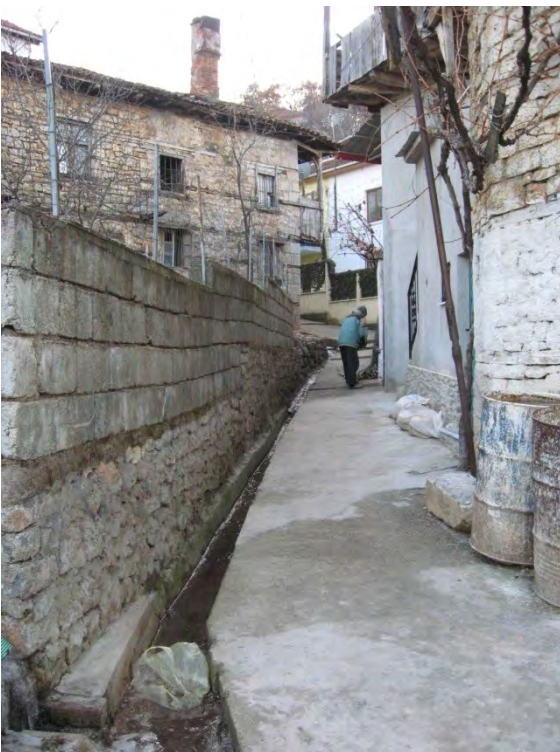
Figure C.42: Rain water channel in Lin (Niebel 2012)
