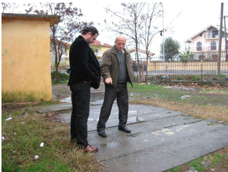
Figure C.21: Vat Gjeloj explains the situation of the school while standing on the “septic tank” (Niebel 2011)
