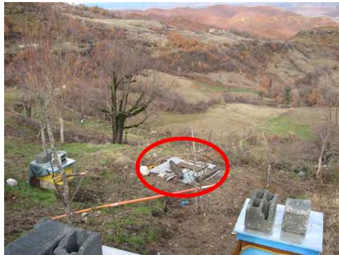
Figure C.33: Shared pit of several families without proper cover fills up while rain (Niebel 2012)
