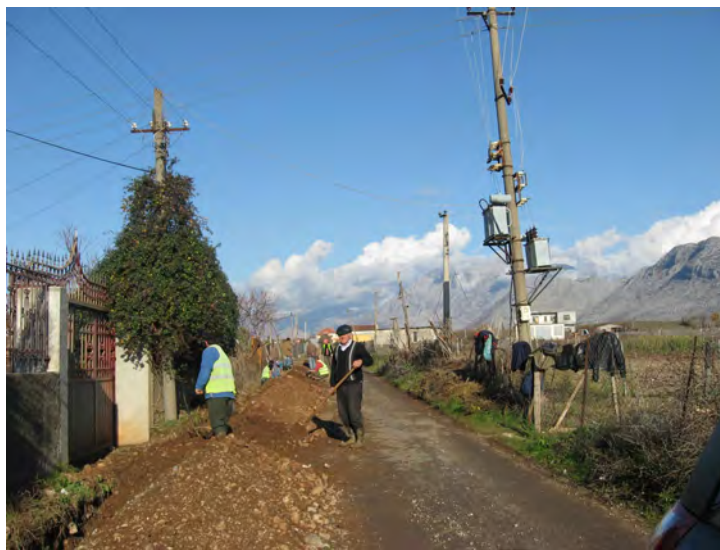
Figure C. 5: Ongoing construction works for the water supply project of ADF (Niegel 2011)
