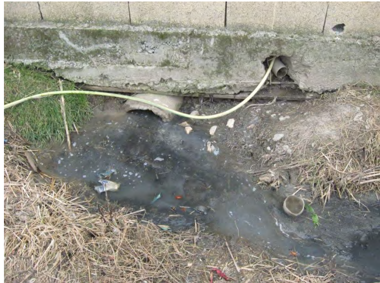
Figure C.57: Black wastewater in the open sewer in Hamallë (Niebel 2012)
