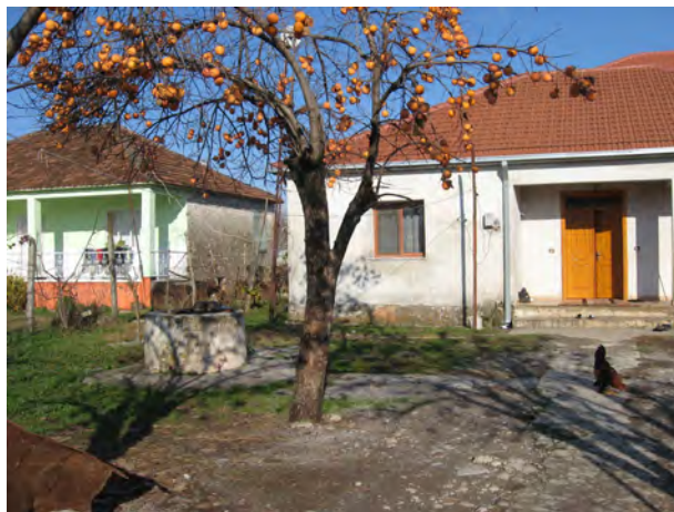
Figure C.4: Houses in Dober (Niegel 2011)
