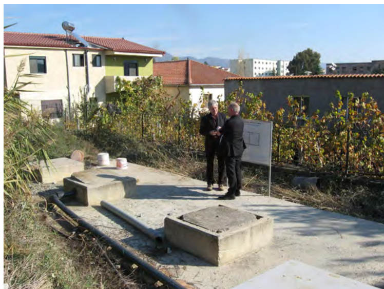
Figure 5.6: Imhoff tank and settling tank at the constructed wetland plant in November 2011 (Niegel 2011)
