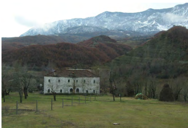
Figure 6.1: House in the commune Gurre (Niebel 2012)
