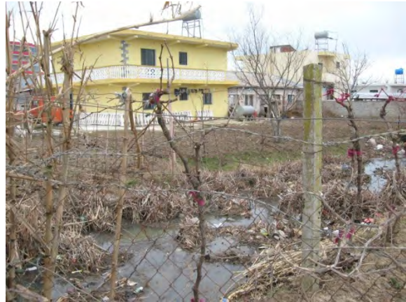
Figure C.55: Wastewater collector in a private yard behind the house in Hamallë (Niebel 2012)
