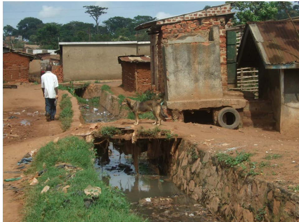
stream / drainage channel
