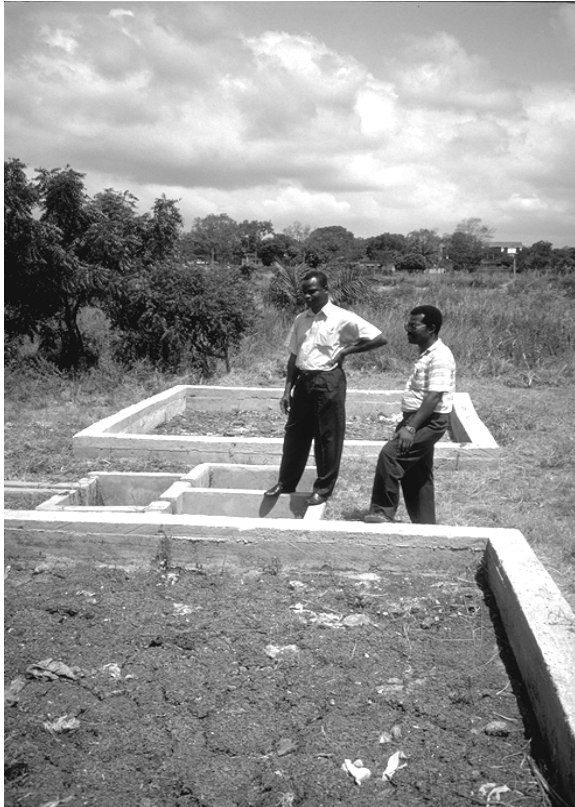
Figure 4 Pilot sludge drying beds in Accra, Ghana
