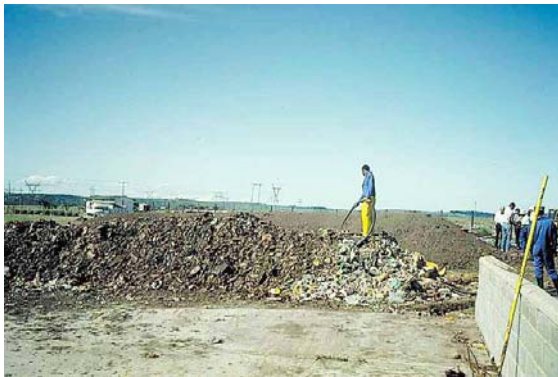
Figure 6 Sprinkling FS over refuse at the Rini/Grahamstown (South-Africa) co-composting plant
