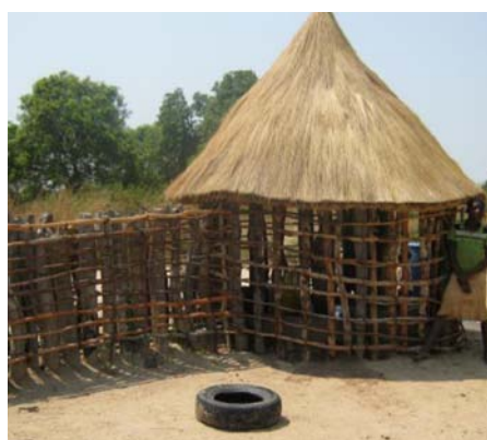
Protection around the water pump to prevent animals from accessing it
