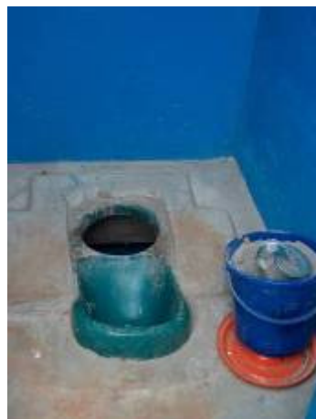
Figure 18: Squatting pan for faeces and urine separation (Kalungu, Uganda).
