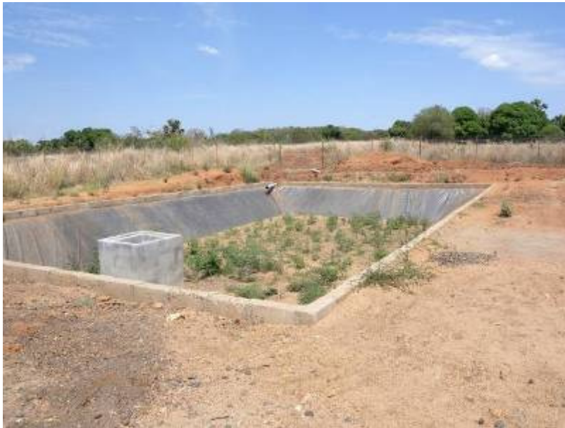
Figure 22: Sludge drying bed for a hospital (Kitgum, Uganda).
