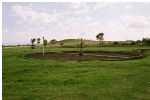
Figure 23: Trickling filter (Nakuru, Kenya).
