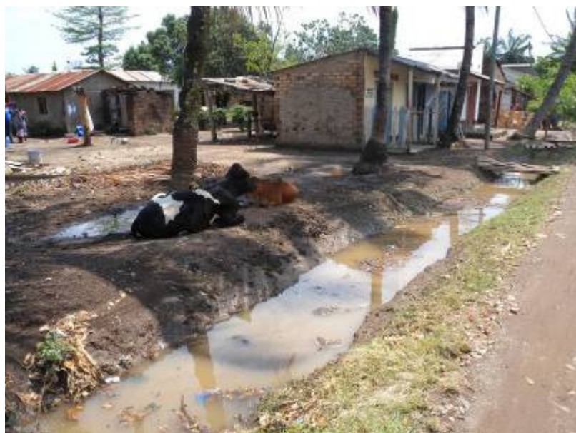
Figure 11: Drainage channel full of stagnant water one day after rainfall.
