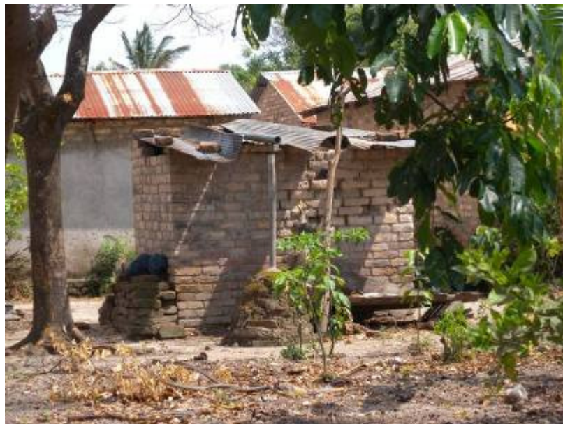
Figure 5: Pit latrine at household level.
