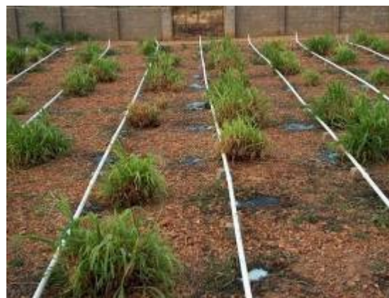
Figure 24: Constructed wetland system (Matany Hospital, Uganda).
