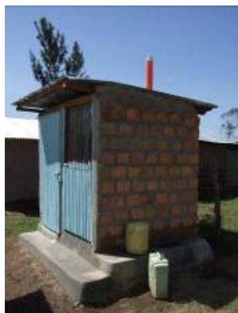
Figure 15: Ventiladed improved pit latrine (Kisumu, Kenya).
