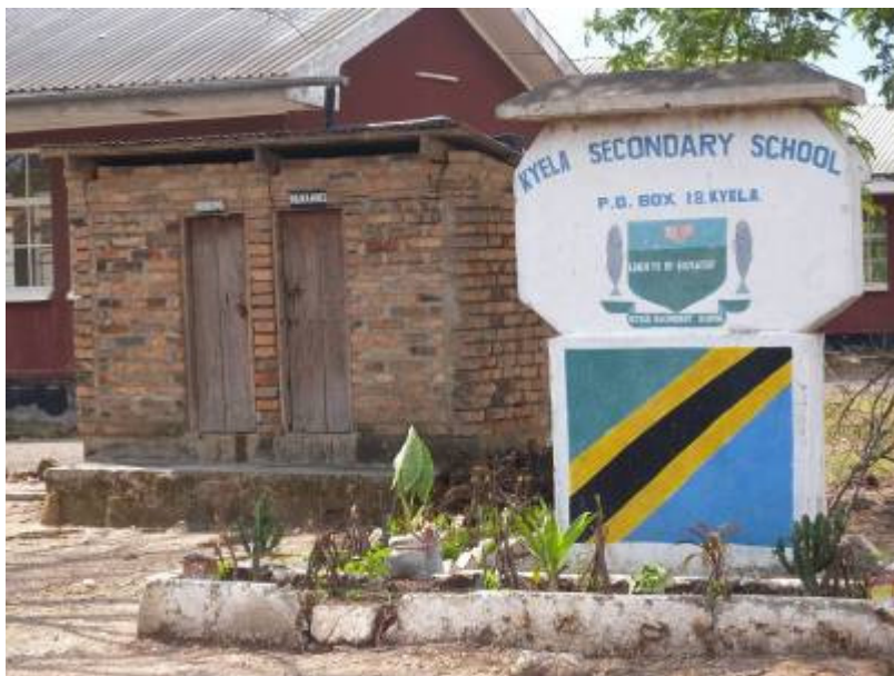
Figure 7: Pit latrines for a secondary school, one for girls and one for boys.
