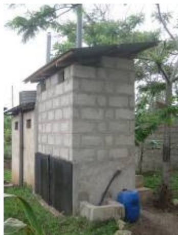
Figure 17: Urine diverting dry toilet (Arusha, Tanzania).
