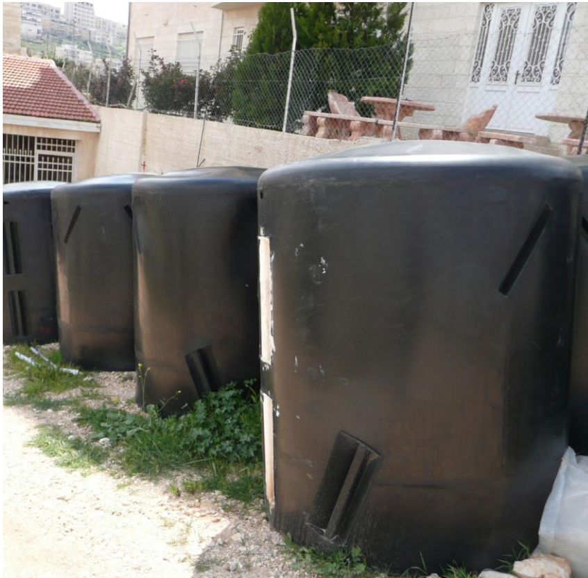
Sewage transfer stations
