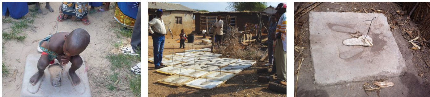
In Tanzania, community-wide events promoted sanitation behavior change and affordable, child-safe options such as the Sungura slab (left). Masons received training in latrine construction (middle) to strengthen the quality and availability of products that consumers preferred and could afford (right).
