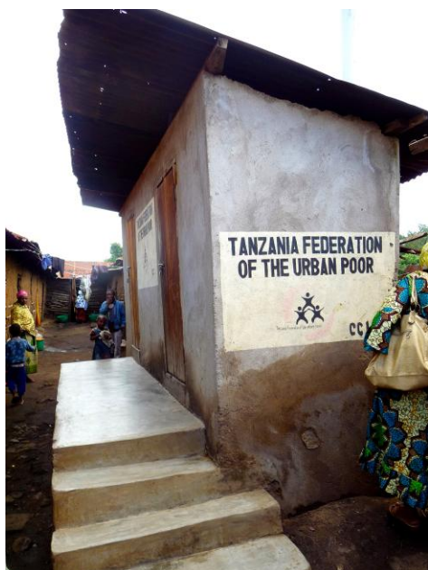
Completed ecosan toilets in Arusha, Tanzania.
