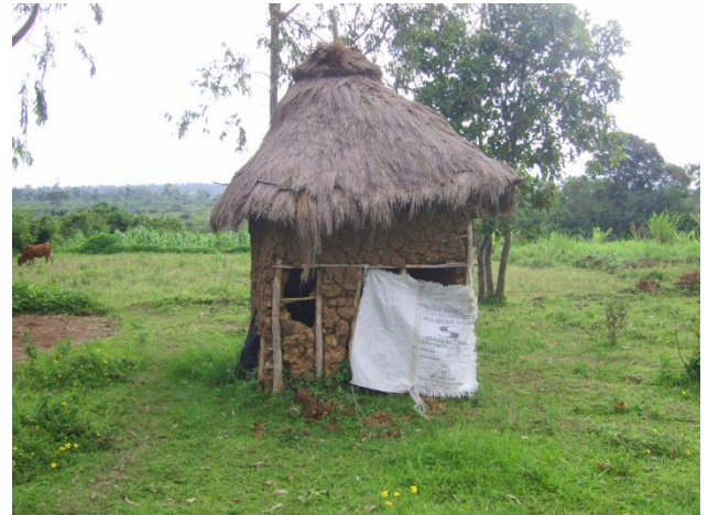
Picture 11: UDDT was unfinished therefore pit latrine was used instead
