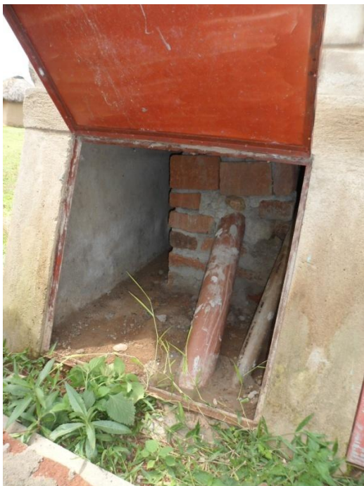
Picture 8 Male beneficiary was not sensitised. He inserted pipes in the dehydration chamber leading to an offset pit
