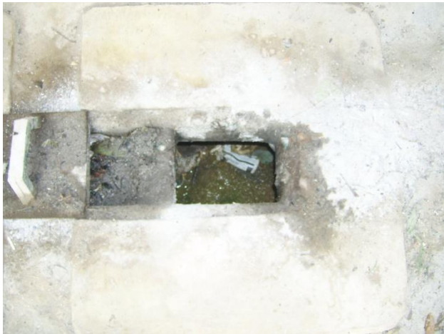
Picture 10: The UDDT used as a pit latrine
