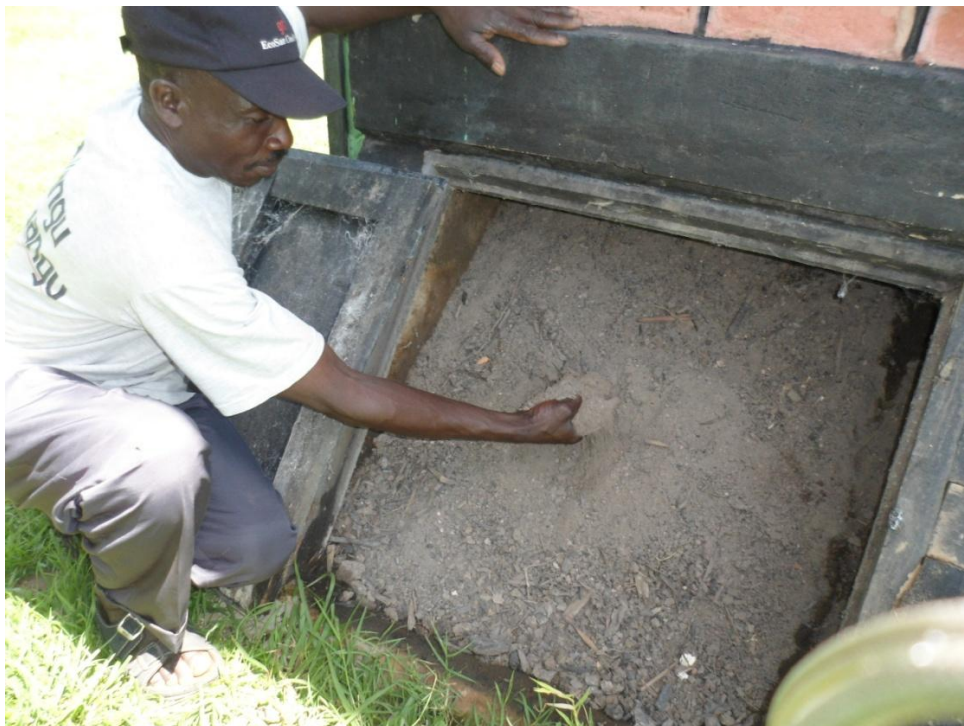
Inspecting the texture of the fertiliser in a dehydration vault
