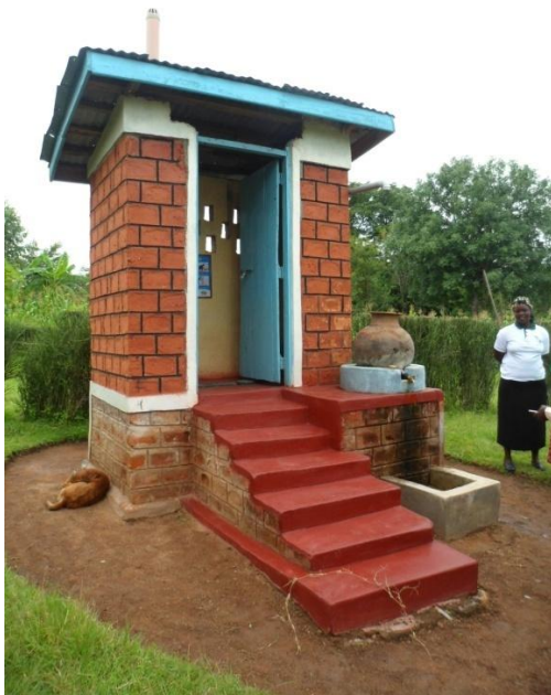
Picture 1: Double vault UDDT
