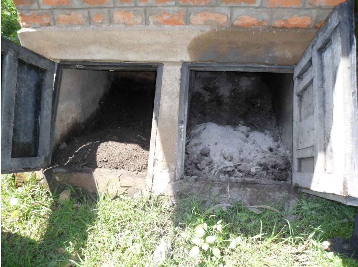
Picture 12: Left: Fertiliser ready for the farm. Right: Dehydrating and sanitisation of the human excreta
