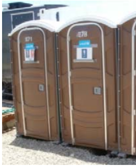
Figure 11. Prefabricated toilets widely used in Port au Prince
