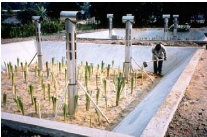
Figure 61. Wetland under construction
