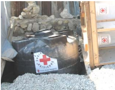
This tank was buried but floated after rain. Note 4 holes in top
