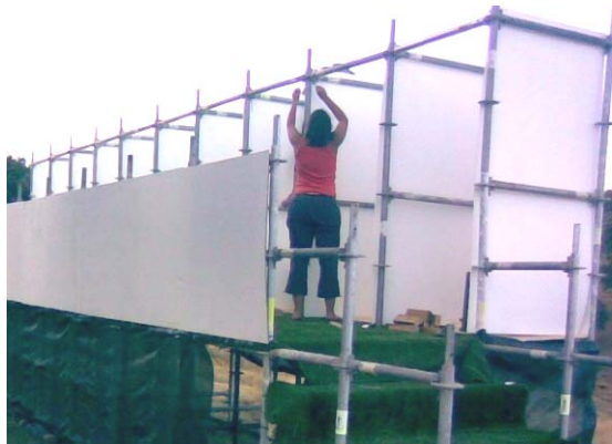
Figure 10. Toilet framework of steel scaffold poles
