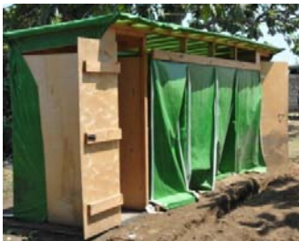
Figure 12. Prefabricated flat packed toilet block installed by IFRC
