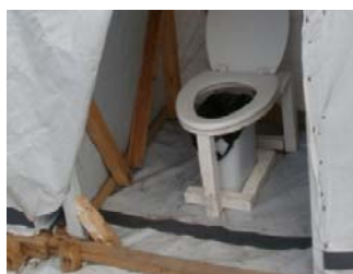
Figure 7. Cubicle floor and walls of plastic sheeting in a single use plastic bag latrine in ?? camp
