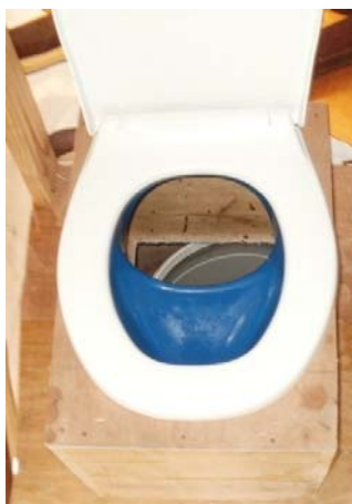
Figure 31. Urine diversion pan
