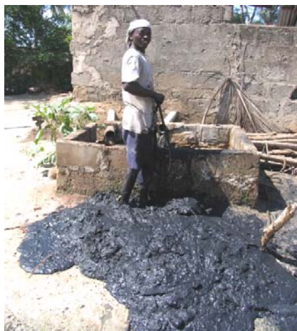
Figure 52. Pit desludging
