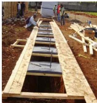
Figure 20. Installing squatting pans over a trench
