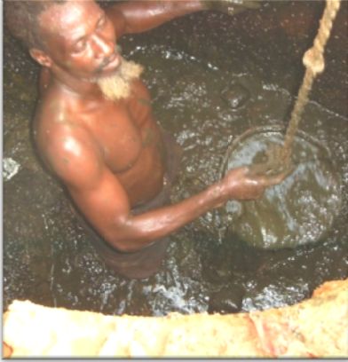
Figure 47. Manually emptying a pit latrine
