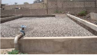
Figure 54. Sludge drying bed
