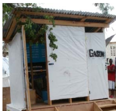
Figure 6. Timber framed door with simple internal lock on a urine diversion toilet in ?? camp
