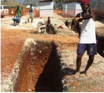
Figure 19. Digging trenches for toilets
