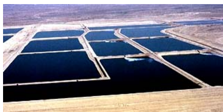
Figure 57. Conventional WSP layout
