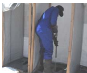
Figure 40. Water jetting to liquefy trench latrine wastes
