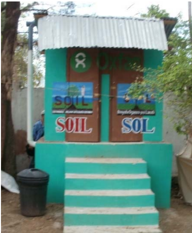
Figure 3. Poor toilet access on a urine diversion toilet in ?? camp
