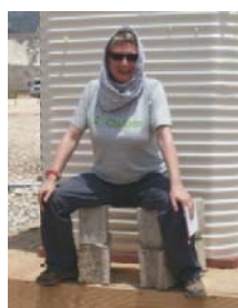
Figure 17. Block pedestal for disabled users
