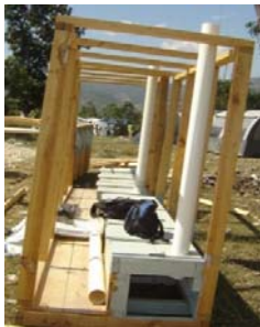
Figure 21. Pedestal toilets for trench latrine under construction
