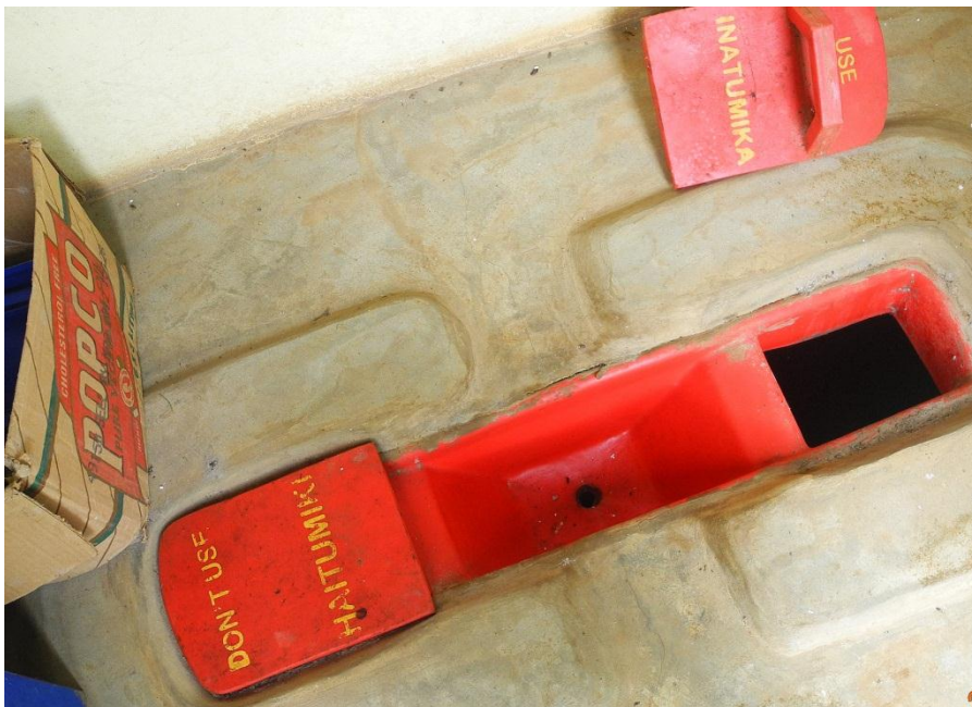
Figure 4, A squatting pan for a double vault UDDT system.
