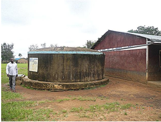
Figure 27, A big water tank for harvested water from the roofs of the main buildings in Khaimba Primary School.
