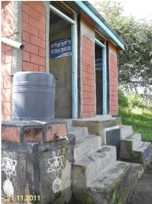
Figure 20, UDDTs for the teachers were mainly in good condition.
