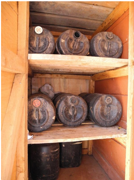
Figure 24, Urine is stored in the containers in a closet by the UDDTs. Containers are labelled by the date and stored for 14 days of minimum before delivering to the farm.
