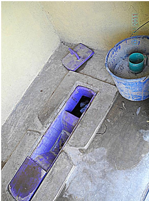
Figure 7, Squatting pan of a double vault UDDT in Kendu Muslim Secondary School.
