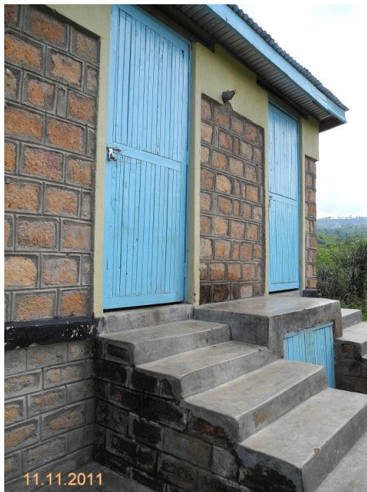
Figure 16, UDDTs for boys in Kachan Primary School.
