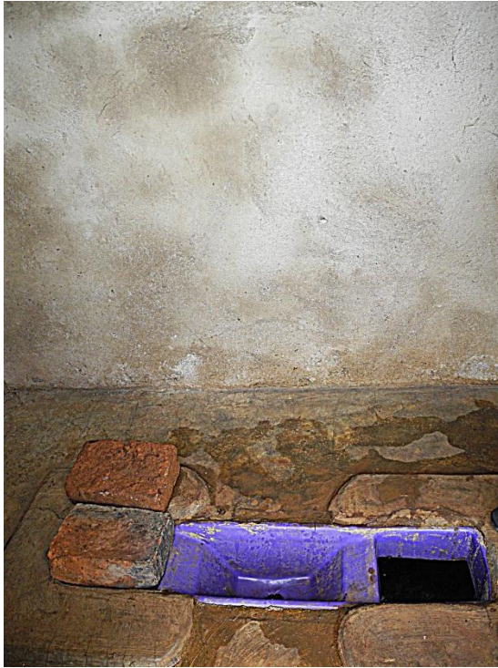
Figure 17, Floor, walls and the squatting pan were clean. The hole for the storing vault was closed with a brick.
