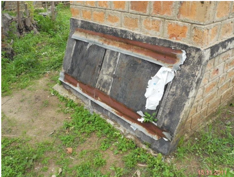
Figure 19, Vault doors behind the UDDT.
