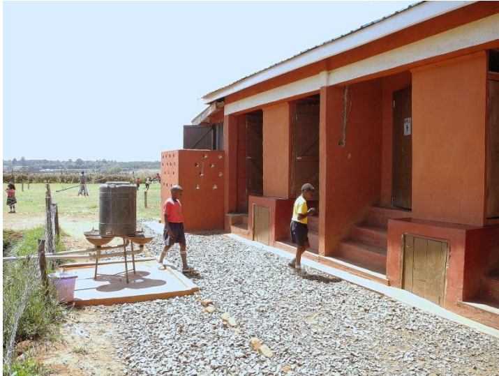
Figure 22, UDDTs in Eldoret Educational Centre are all built in one unit. There are two UDDTs for girls, one for teachers and one for boys. In addition there is a urinal for boys. On the left is the hand washing tank with four taps.
