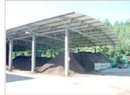
Compost store house Anaerobic digestion facility, Passau
