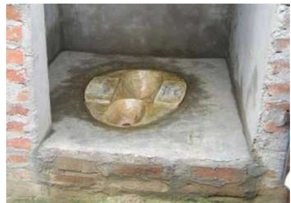
Fig. 6: Urine diversion squatting pan in Sabaithuwa village. Anal washwater is collected together with faeces (source: Heijnen, 2006)
