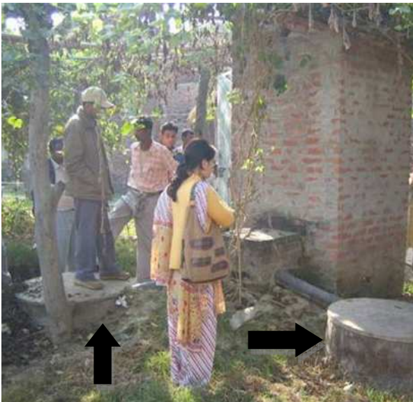
Fig. 5: Double-pit urine-diversion latrines in Sabaithuwa (source: Heijnen, 2006). The black arrows point to two pits which are offset from the toilet house.
