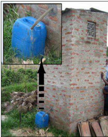
Fig. 8: Urine collection in 20-L jerricans behind the toilet in Sabaithuwa village (source: Heijnen, 2006)
