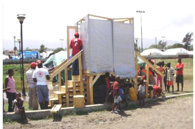
Figure 1: Raised toilets in Haiti provided by IFRC for 275,000 people per day with materials produced in Dominican Republic and constructed in Haiti (source: Spanish Red Cross, 2010).
