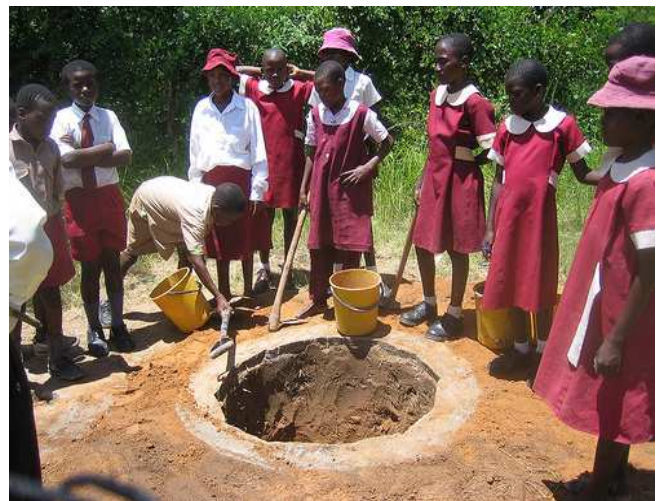
Figure 1: Pupils at a school in Epworth, Harare in Zimbabwe learn to build their own toilets: digging the shallow pit of an Arborloo inside a concrete ring beam (source: Aquamor, Zimbabwe, 2009). More photos of this school available here: www.flickr.com/photos/gtzecosan/sets/7215762630000229/
