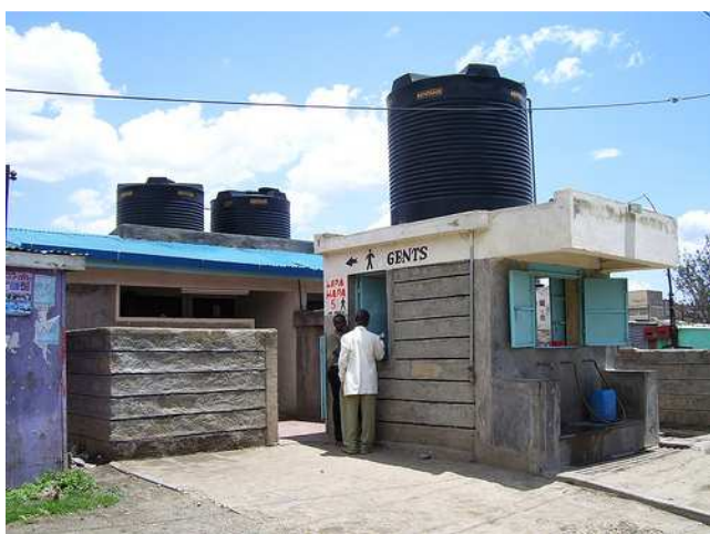
Figure 6: Naivasha public toilet with water kiosk. In front is the water kiosk that functions as an operator room. Customers pay at the side window, where the two people are standing. Behind them the gents section of the toilet can be seen (source: C. Rieck, 2008) 3 .
