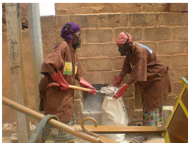
Figure 1: Two staff members from a service provider are emptying the faeces vaults of household UDDTs in Ouagadougou, Burkina Faso (source: S. Tapsoba, 2009) 1 .
