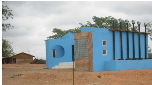
Figure 4: The Baranuka High School (in Lulekani, South Africa) toilet block that was built by The Clean Shop and Trevor Mulaudzi and serviced by the school (source: T. Mulaudzi, 2008)
