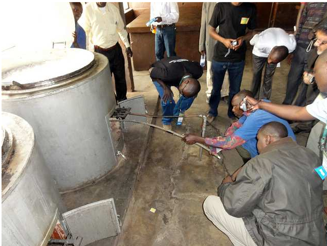
Figure 6: A stove in a school kitchen running on biogas produced from human excreta in Rilima, Rwanda (source: P. Feiereisen, 2011). More photos on this school: www.flickr.com/photos/utzecosan/sets/72157627230220319/with/6008002835/ .
