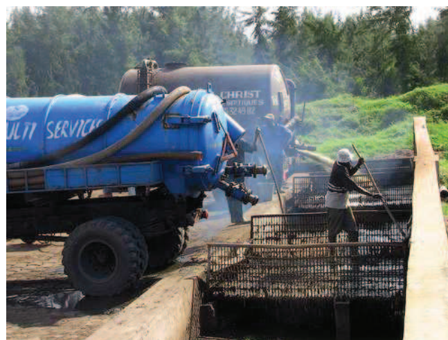
Figure 4: Faecal sludge being discharged from trucks into treatment beds in Cotonou, Benin (source: S. Blume, 2010).
