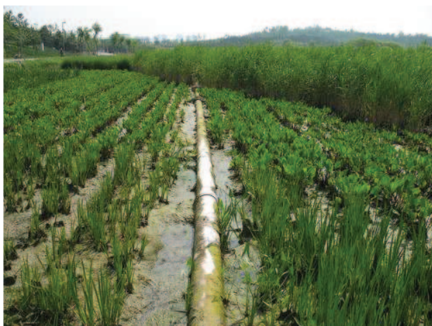
Figure 3: Vertical flow constructed wetland in the “Olympic forest park” located north of the city centre of Beijing, Peoples Republic of China, 2008 (source: J. Germer, 2008) 4 .
