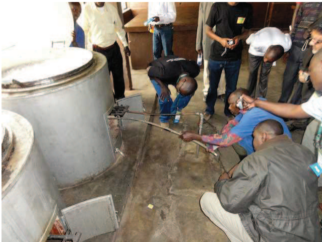
Figure 6: A stove in a school kitchen running on biogas produced from human excreta in Rilima, Rwanda (source: P. Feiereisen, 2011). More photos on this school: www.flickr.com/photos/qtzecosan/sets/72157627230220319/with/6008002835/ .
