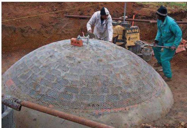
Figure 5: Construction of a fixed dome biogas plant, Lesotho (source: M. Lebofa, 2006).
