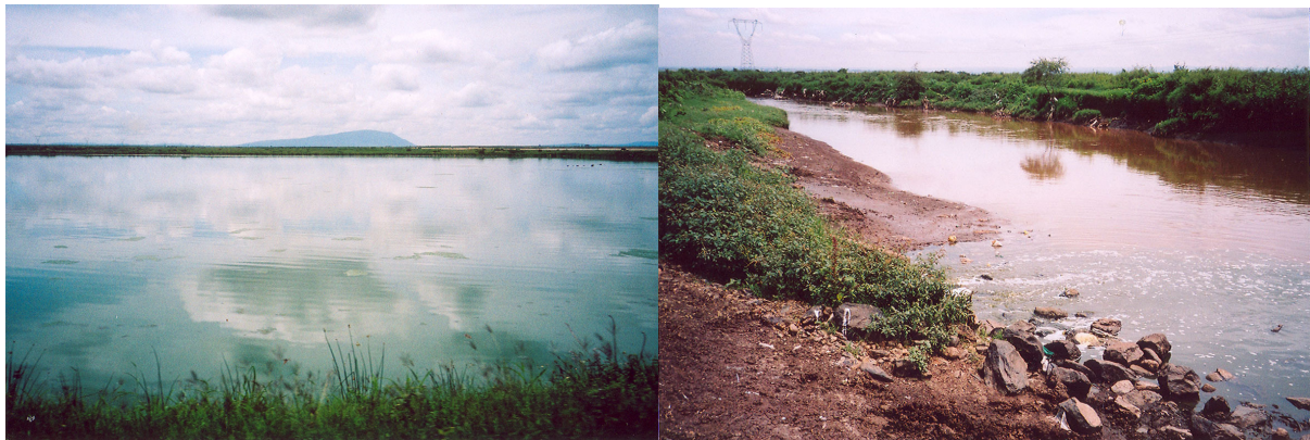
Figure 32: Facultative pond of the Dandora treatment pond system and discharge into the Nairobi River
