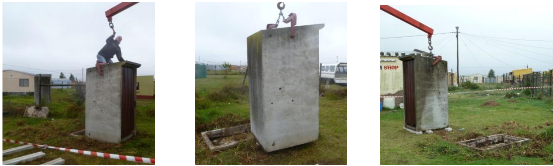
Figure 3 the process of lifting the unit with the crane
