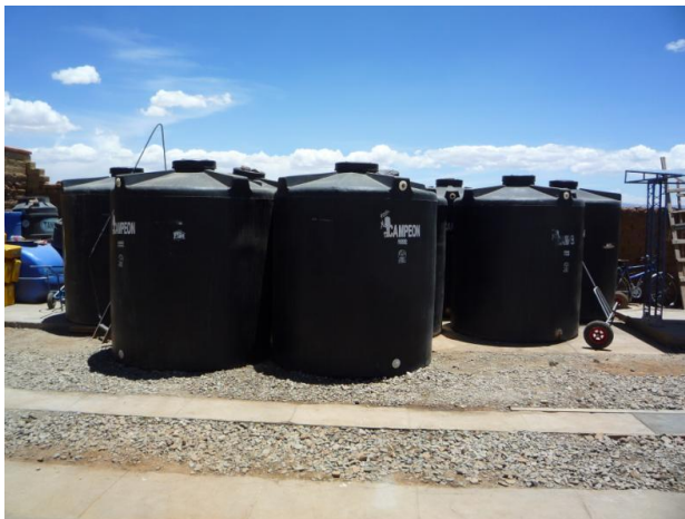
Fig. 7: Storage of urine at the composting centre in 5,000 L plastic-tanks (Andersson, 2011).
