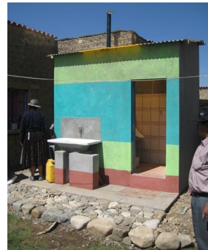
Fig. 8: Front view of the UDDT unit with handwash basin on the outside (Andersson, 2011).
