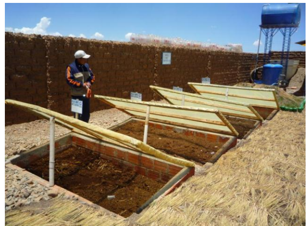
Fig. 6: Composting trenches for treatment of the faecal matter (Andersson, 2011).
