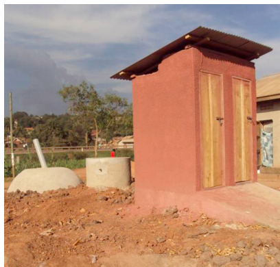
Bio-latrline constructed in Mulago III
