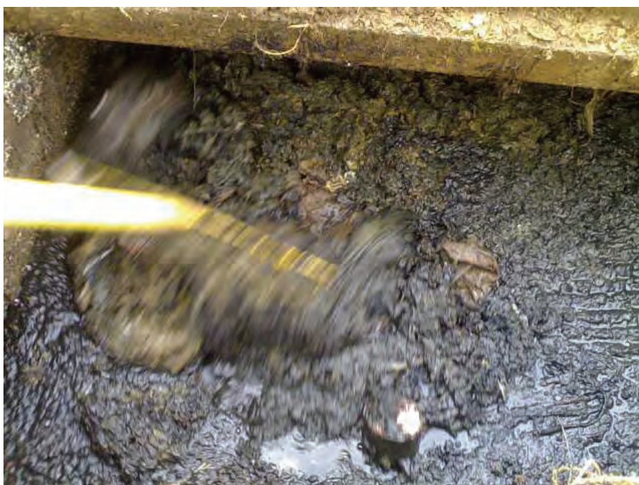
Removing rubbish from a pit with a rake prior to emptying
