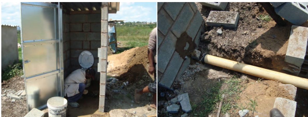
Figure 4.18 Household 4: A structure was built for Household 4 to house the pourflush toilet.
