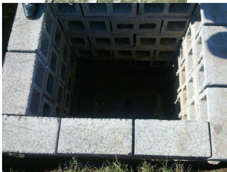
Figure 4.23 Top structure (left) built for church with soak pit collecting some water (right)
