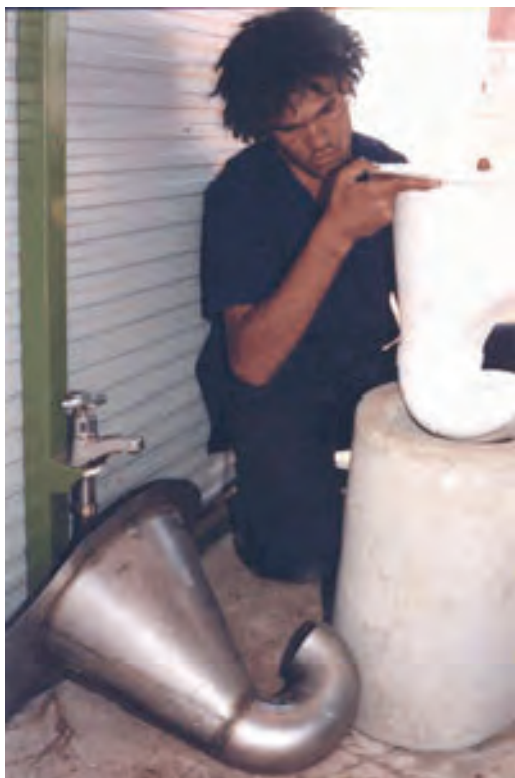
Figure 2.12 Australian pour flush pedestal (RADG, 2003)
