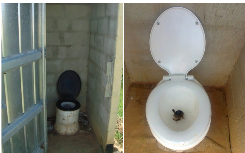
Figure 4.21 Household 7: Previous VIP toilet (left) converted to pourflush (right).
