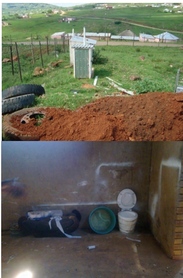
Figure 4.22 Household 8: Two existing VIPs and digging of soakpit (left). VIP installed in garage where animals are also kept; owner intends to enclose part of the garage as a bathroom (right).
