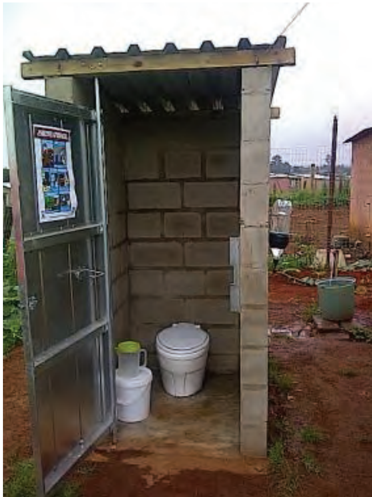
Figure 4.14 Outdoor structure with pour flush pedestal. A handwashing facility is mounted on the right hand side of the structure. The bucket and jug for flushing are stored in the loo and a poster explaining how to use and care for the system is mounted on the inside of the door
