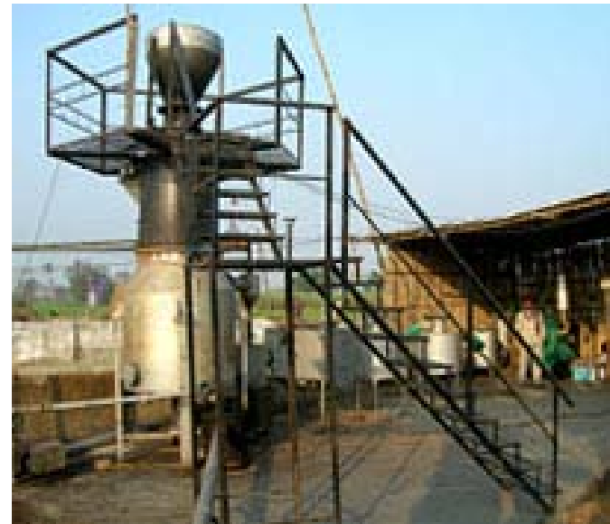
Husk Power's rice husk gasifier
