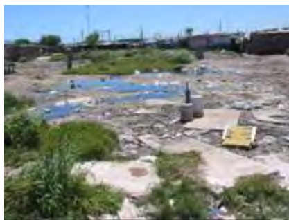
Kosovo, 2005. Greywater problem around standpipe
