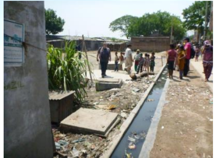
Biogas septic tank in Dhaka, built by "Practical Action", 10 years ago
