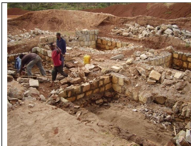
Figure 3-9 c. Improved official dumping site under construction
