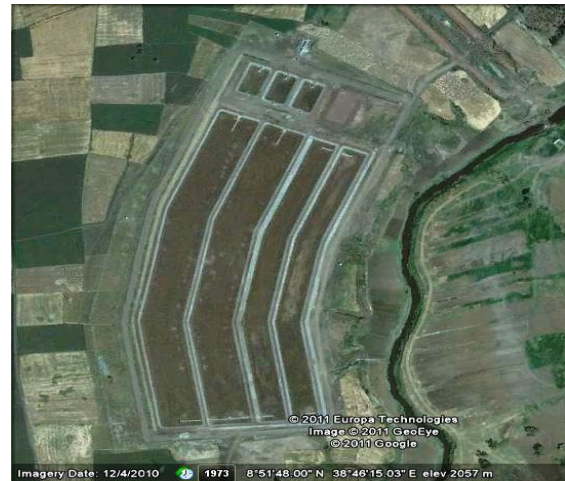
Figure 3 6 Gelan WWTP -Stabilization ponds
