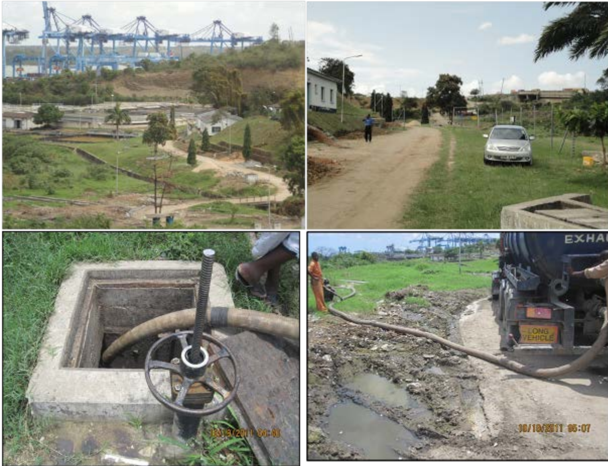
Figure 3-11 : Kipevu WWTP (TL), Access (TR), disposal point (BL), Truck emptying
