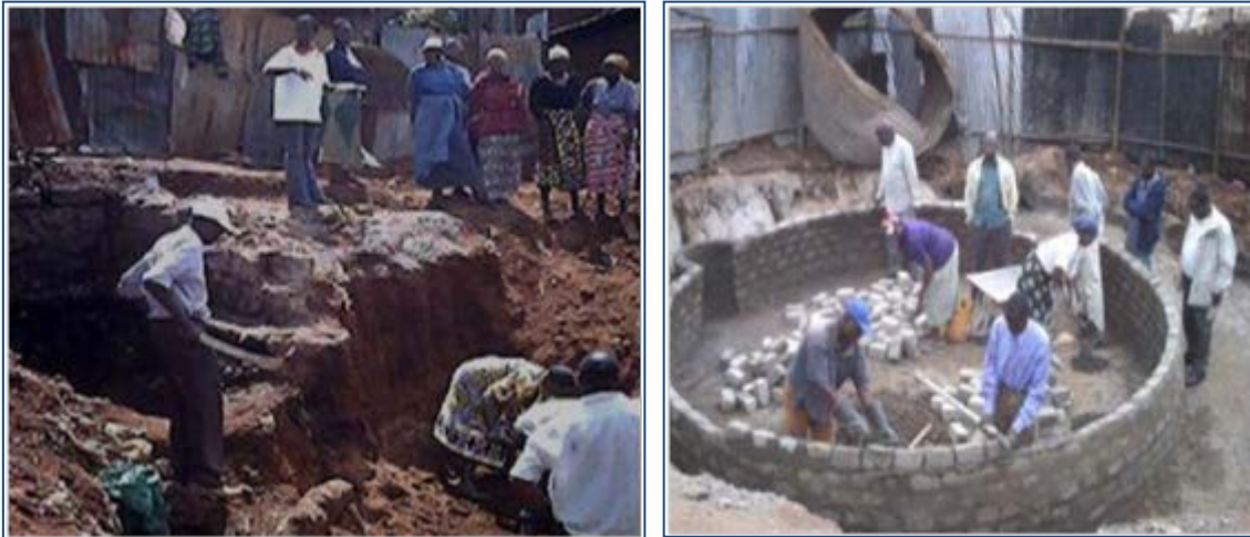
Figure 3-35 : Excavation and Laying of Foundation for Bio-Centre
