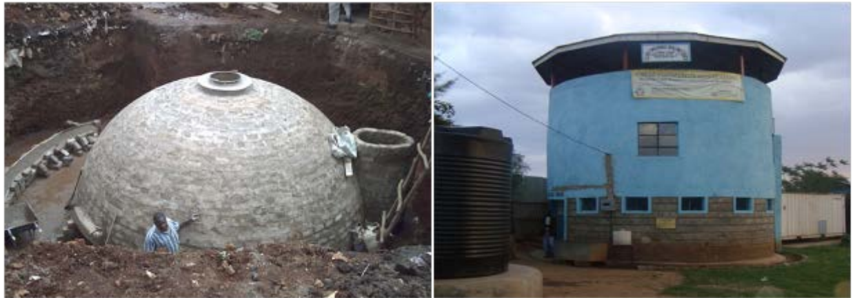
Figure 3-33 : Construction of Bio- center; Kisumu (left); Stara Bio-centre; Nairobi
