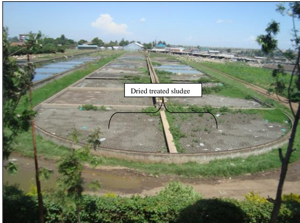
Figure 3-40: Second sludge drying bed at Kariobangi Treatment Plant
