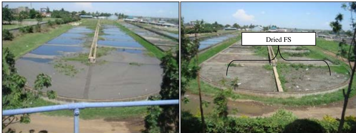
Figure 3-25 : FS Drying Beds - Kariobangi WWTP Nairobi
