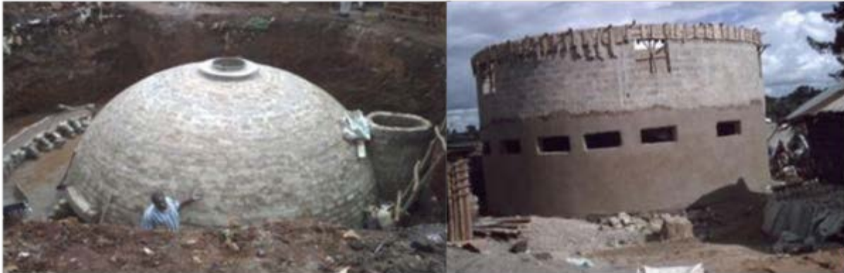
Figure 3-36 : The dome and super structure of a Bio-centre
