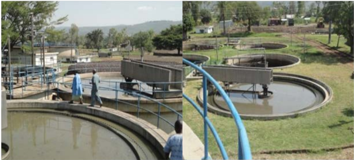
Figure 3-23 Sedimentation Tanks at the Kisat Wastewater Treatment Plant
