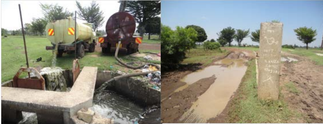
Figure 3-8 : FS Disposal at the inlet of Nyalenda TP (left) and access to the plant (right)
