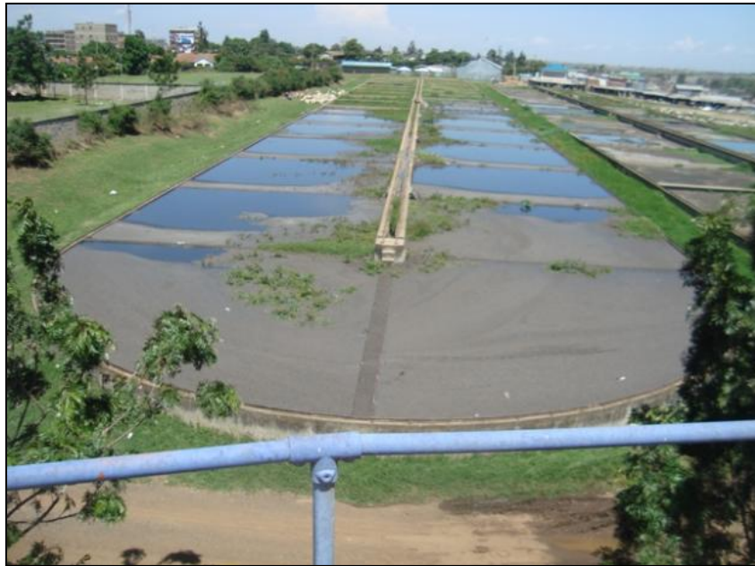
Figure 3-39: First sludge drying bed at Kariobangi Treatment Plant
