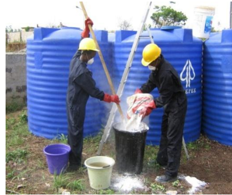
Figure 2 Fecal sludge management using lime (Sridhar 2010)
