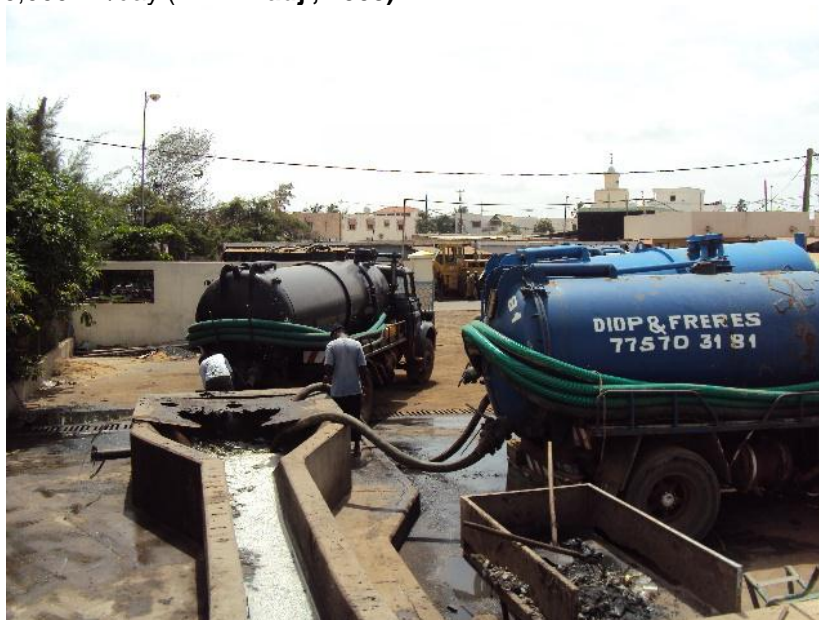
Figure 9: Sludge trucks discharging at the Cambérène FSTP
