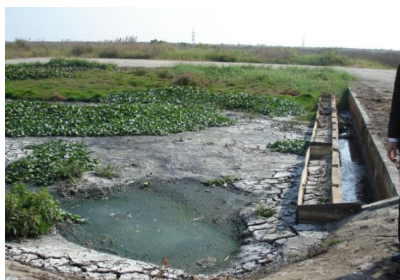
Figure 4-54. Settling pond for FS treatment in Trang Cat
