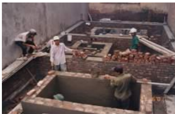
Figure 4-14. Construction of septic tank in urban area of Hanoi
