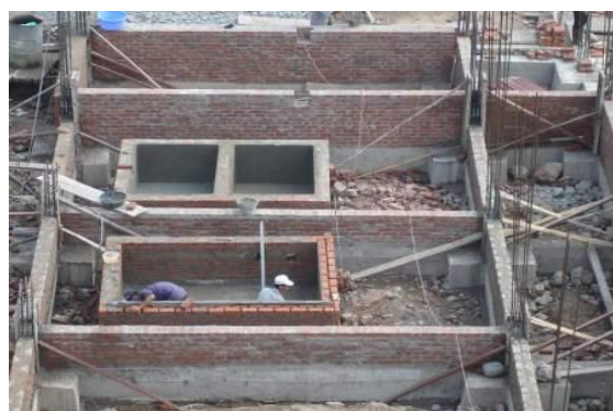
Figure 4-14. Construction of septic tank in urban area of Hanoi
