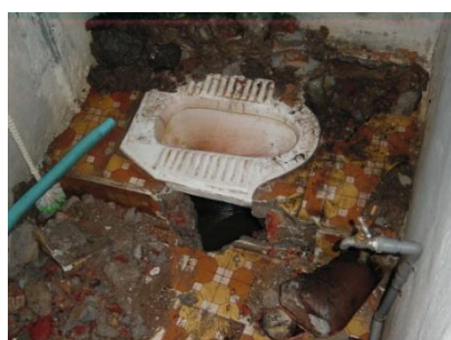
Figure 4-51. Floor breaking for desludging
