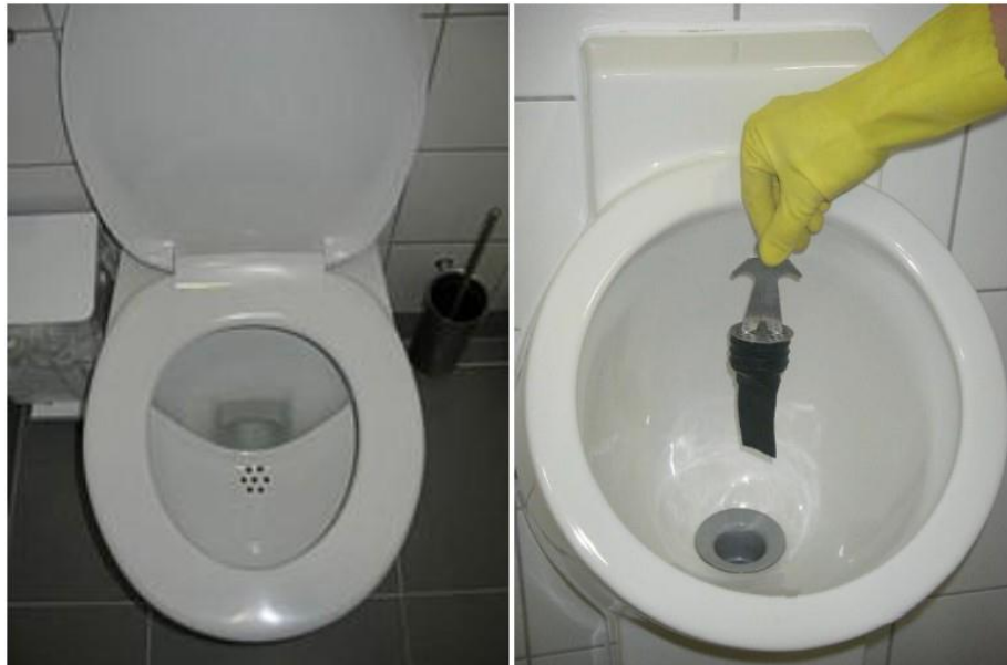
Figure 2 NoMix UD toilets (right) and waterless urinals (Source: Hartmann, 2011)
