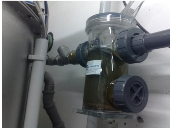
Figure 13 Basket strainer in front of MAP reactor
