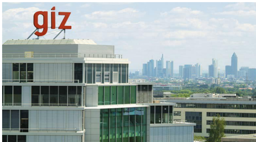
Figure 5 The main building (“House 1”) at the GIZ headquarters in Eschborn near Frankfurt, where this project is implemented (Source: GTZ, 2009).
