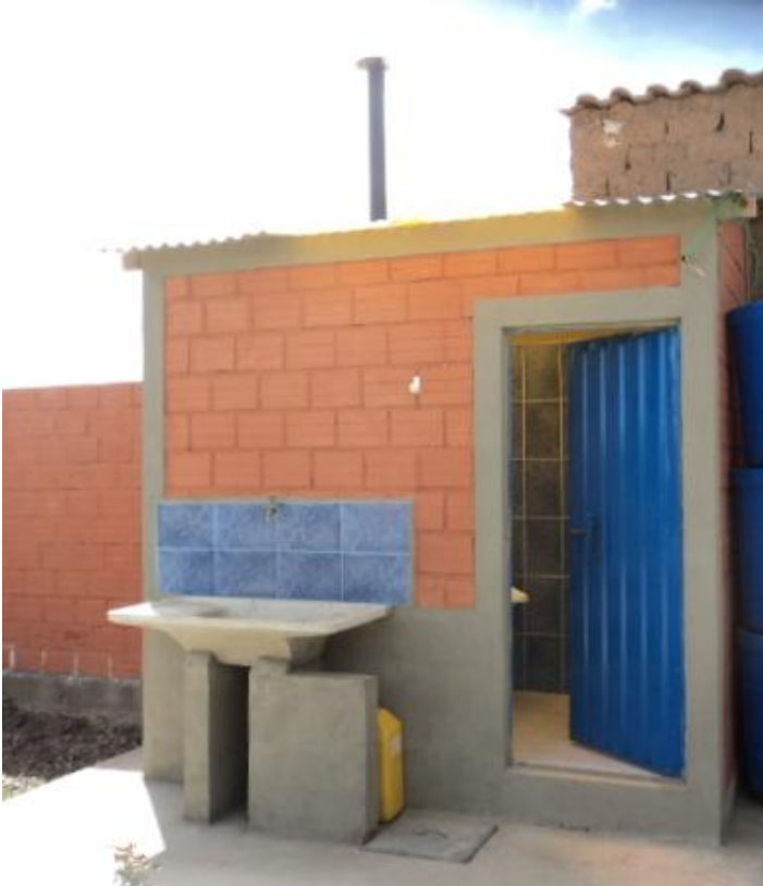
P.1 A one door Ecological toilet model in District 7. 8
