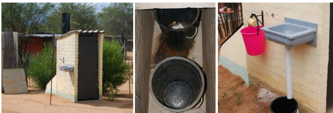
Fig. 2: Left: Otji toilet in Omaruru; Middle: Perforated faecal containers in the vault; Right: Basic handwash basin attached to the toilets. The pink bucket provides fresh water, the cup is used to fill the basin and the black bucket collects the greywater which can be used for irrigation (photos: F. Kleemann, GIZ, 2011).
