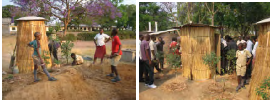
The area around the new pit and its circle of trees is levelled off. The newly planted trees and the toilets are inspected by government officials and staff of the Ministry of Health.
