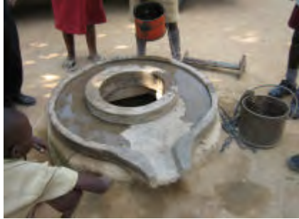
The new well apron is set in position so that the water run-off channel will carry water slightly down hill to a seepage area planted with a tree
