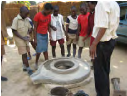
The new well apron is set in position so that the water run-off channel will carry water slightly down hill to a seepage area planted with a tree
