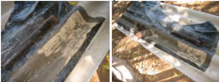
The hessian cement water run-off channel 1.5m long
