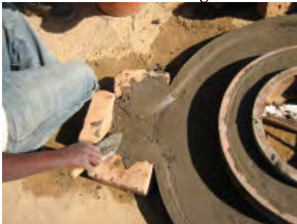
An extension to the apron is made on one side to allow water to flow off into the water run-off channel.
