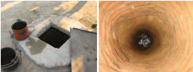
Views of the original well head and down the well chamber
