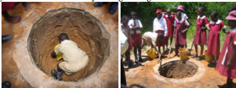
Pit being dug down to one metre depth and soil rammed around the ring beam
