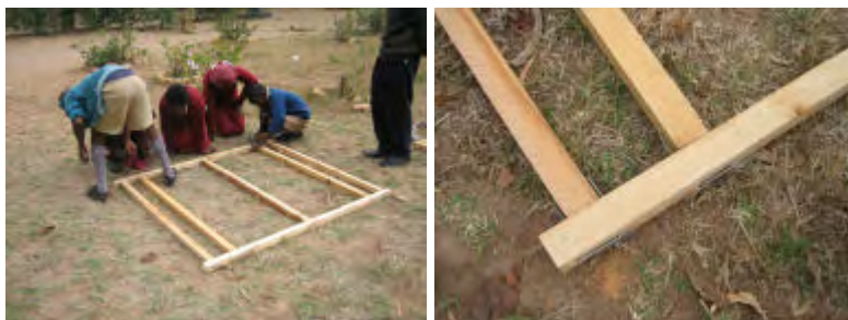
Making the roof frame
