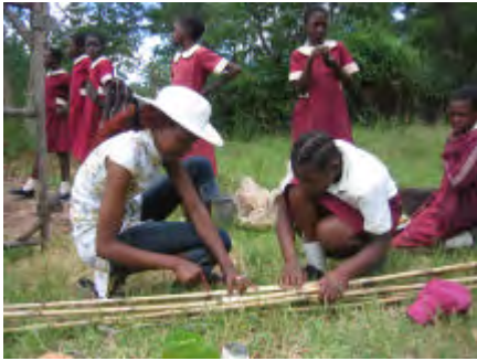
The pupils are also given lessons on how to make vent pipes from reeds and cement and other methods (see in another part of this book for details). A suitable pipe is fitted over the vent pipe hole and through the roof.
