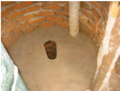
The interior of the Blair VIP toilet showing the cement pipe fitted to the vent hole in the slab and how it passes through the roof.
