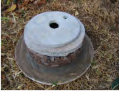
The slab has been added and hole enlarged to suit the urine diverting device used. A miniature urine diverting pedestal is shown.
