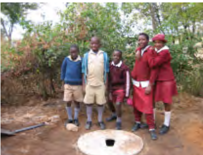
Slab fitted ready for toilet house
