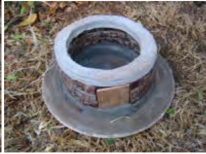
The low brick vault wall has been built on a ring beam. A second ring beam has been fitted on the brickwork and vault access door added.
