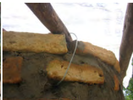
The roof timbers are secured with wire which passes through the brickwork and over the roof poles.
