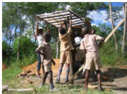
The roof timbers are secured with wire which passes through the brickwork and over the roof poles.
