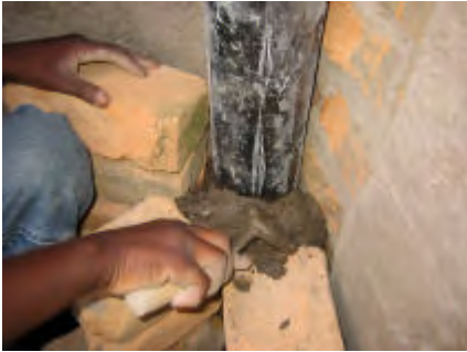
The mortar fills the space between the bricks and pipe. On the right the pipe is almost complete.
