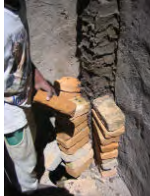
The bricks are then removed from the plaster pipe
