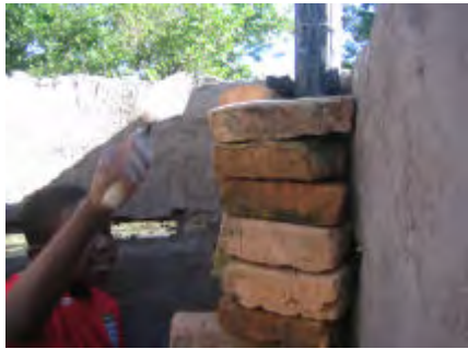
The mortar fills the space between the bricks and pipe. On the right the pipe is almost complete.
