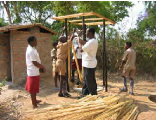
Bundles of grass are built up as walls for this toilet.
