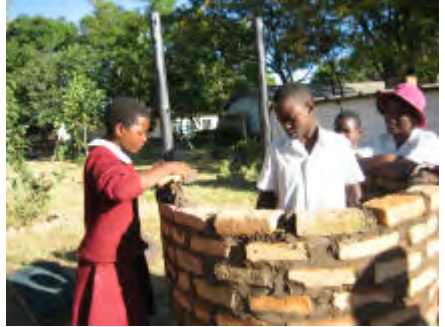
Photos showing the arrangement of the bricks and the bonding technique used.
