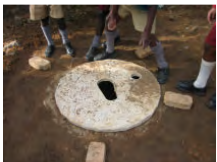
Slab fitted ready for toilet house
