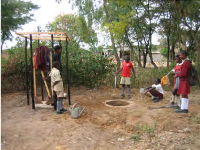
General view of Fossa alterna with two pits and a single structure
