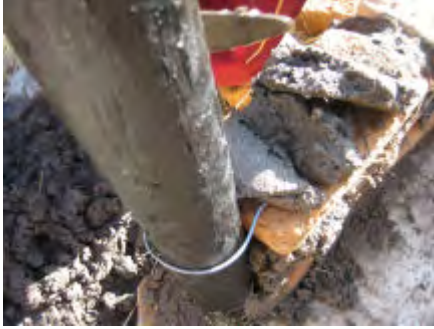
Wire loops can be placed around the poles and into the cement mortar every 5 courses up. These help to bond the brickwork to the poles.
