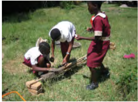
The pupils are also given lessons on how to make vent pipes from reeds and cement and other methods (see in another part of this book for details). A suitable pipe is fitted over the vent pipe hole and through the roof.
