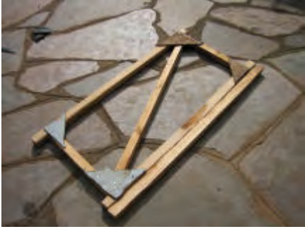
The door frame is made with wooden “brandering” and triangular plywood corners. A single diagonal strut supports the frame. Some form of covering is added to the frame. In this case sacking material called hessian.
