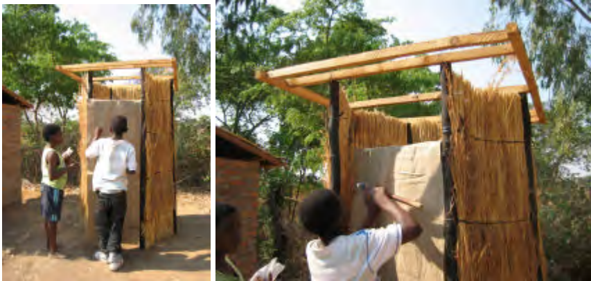
The hessian door panel is nailed to the door frame. This could be treated with cement paint later to make it more durable.
