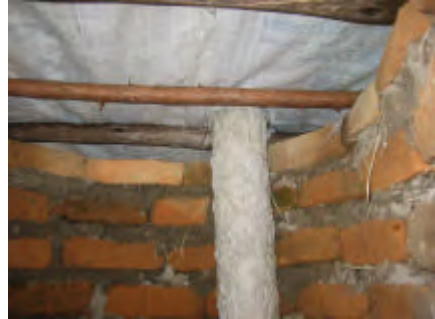
The interior of the Blair VIP toilet showing the cement pipe fitted to the vent hole in the slab and how it passes through the roof.
