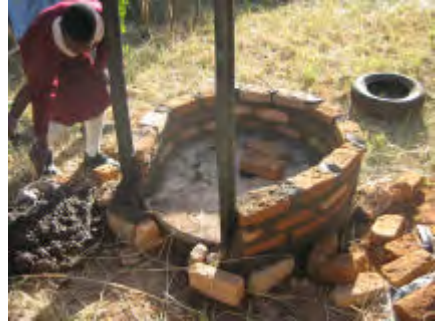
Wire loops can be placed around the poles and into the cement mortar every 5 courses up. These help to bond the brickwork to the poles.
