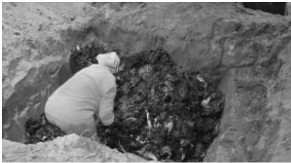
Alternative sludge disposal option: burial on-site.
