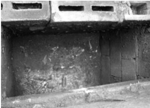
Pit opened for emptying
