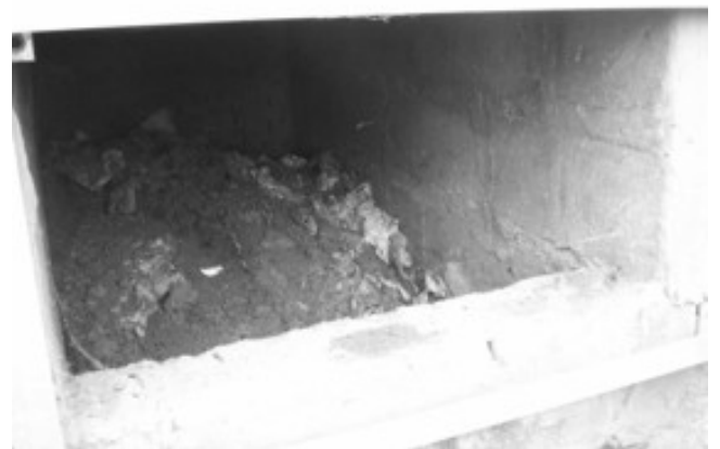
View into a half-filled vault of a double vault urine diverting VIP. The vault is mostly above ground.
