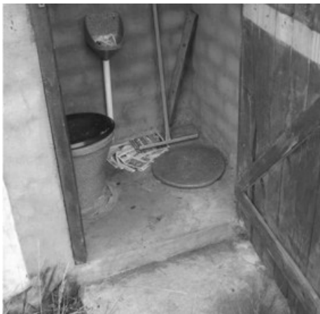
Interior of superstructure. The pedestal contains a urine diverting section for women. Men use the urinal seen on the back wall. The lid of the second vault can be seen at the right of the superstructure interior.
