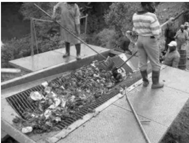
Solid waste remaining on the grids after spraying faecal sludge through the grids
