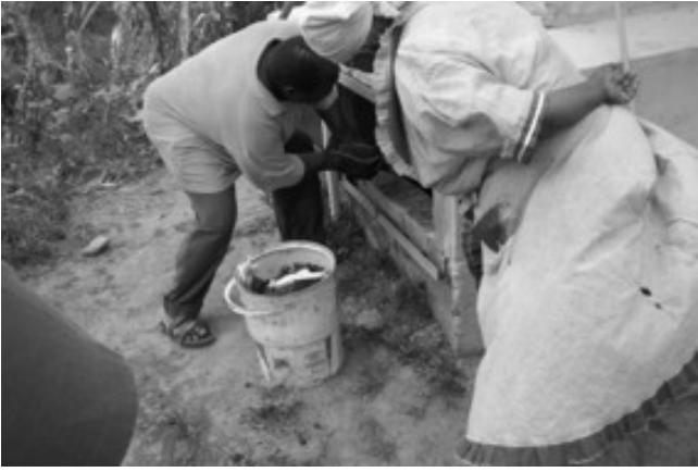
Householders emptying a urine diverting VIP. Householders are encouraged to bury the vault contents on-site.
