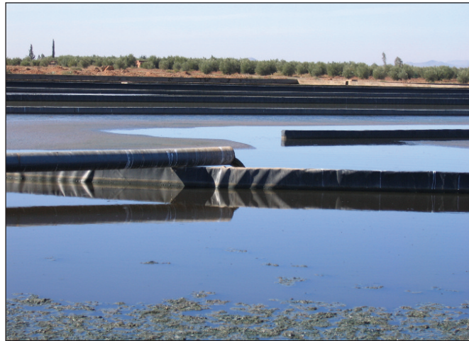
Inlet to high rate algae pond — system overloaded (2006)
