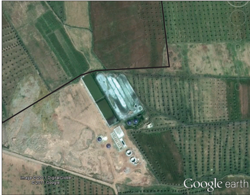
El Attaouia WWTP and zone irrigated with treated wastewater
