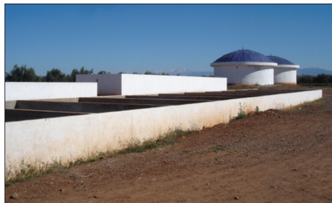
El Attaouia waste water treatment plant — Phase II construction (2011)
