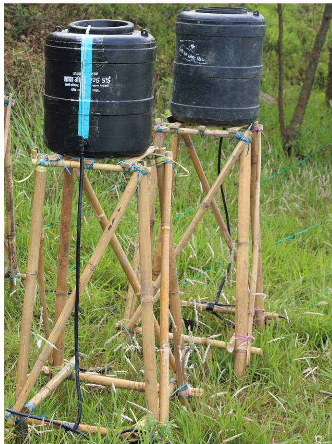
Figure 5: Tank with main line.
