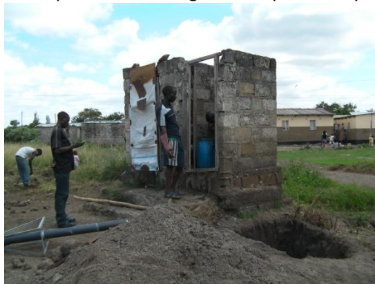
Figure 1: Hole dug next to pit latrine
